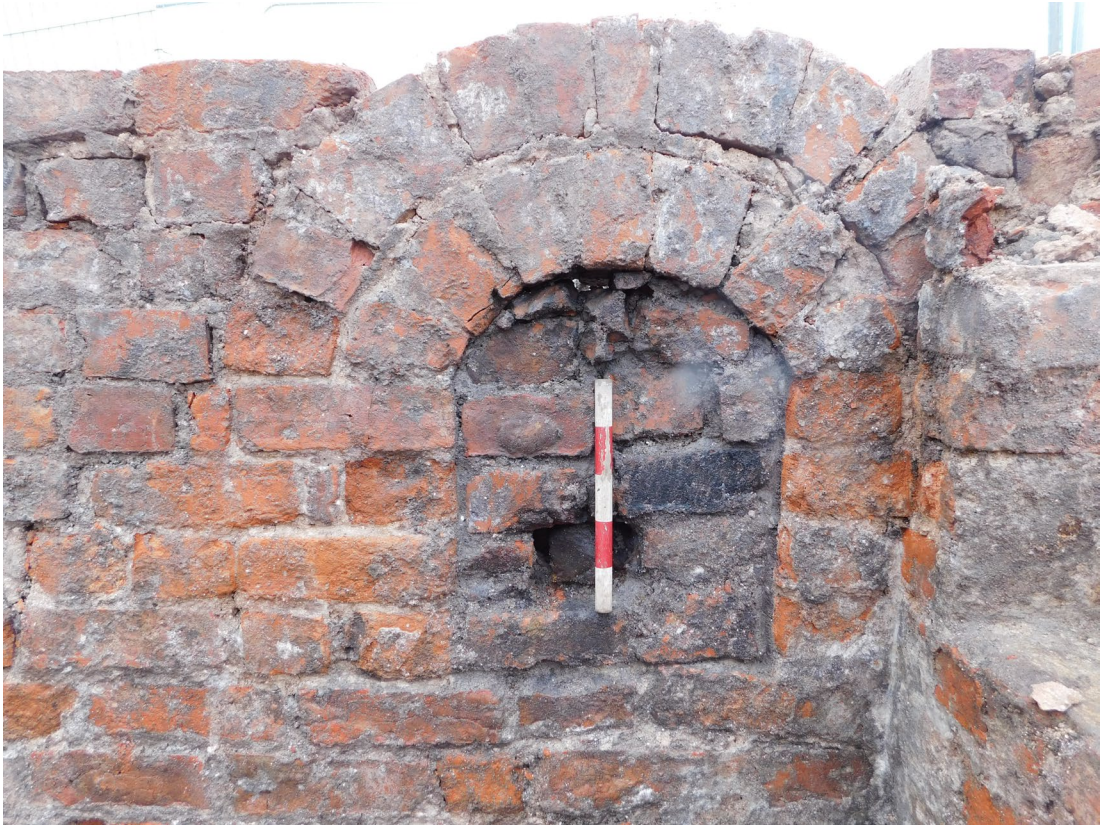
Plate 23: Detail of the arched opening and later blocking (0.25m scale)
