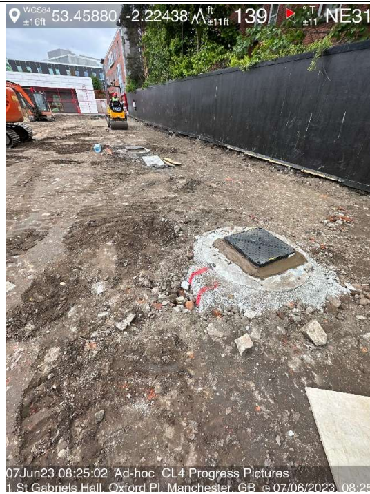
Plate 23: June 7 th , pipe inspection hole.
