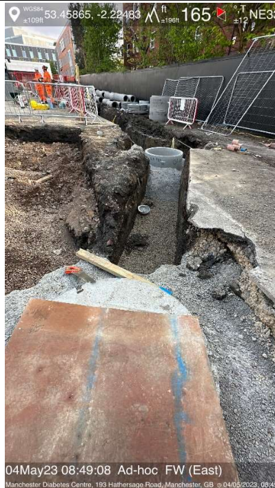
Plate 3: May 4 th , utilities trench with some stone partially filling it.
