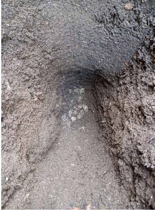
Plate 3: Look downhole at MTP101, displaying concrete and stone at the base.
