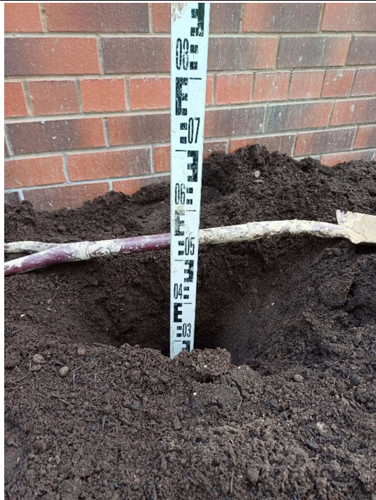
Plate 1: Depth check at MTH101, displaying a clean cover depth of 530 mm.
