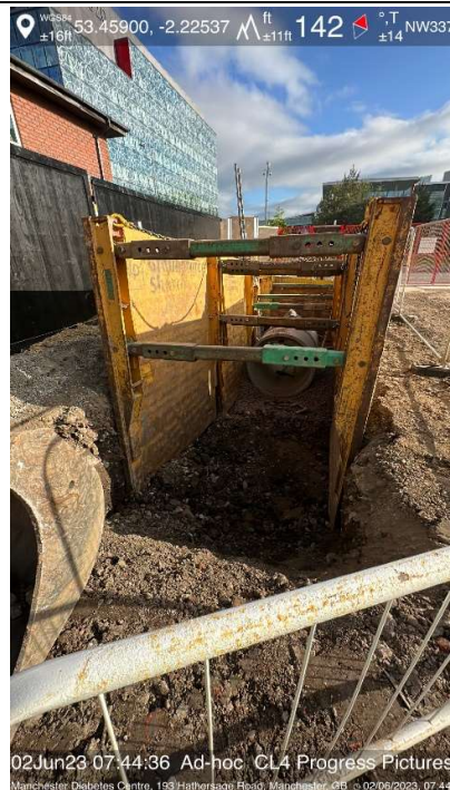
Plate 20: June 2 nd , re-enforced utility trench.
