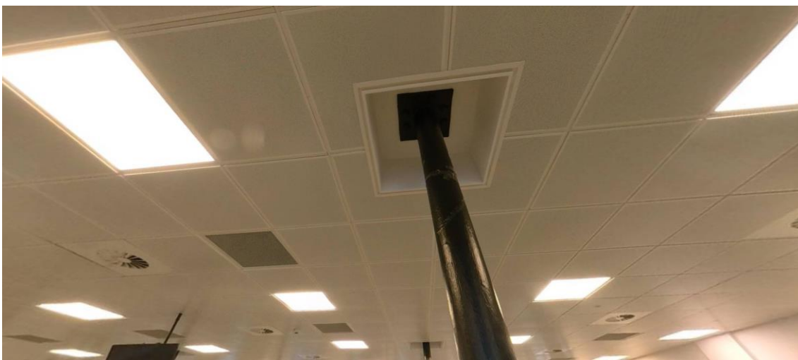
Plate 17: Column recess through suspended ceiling.
