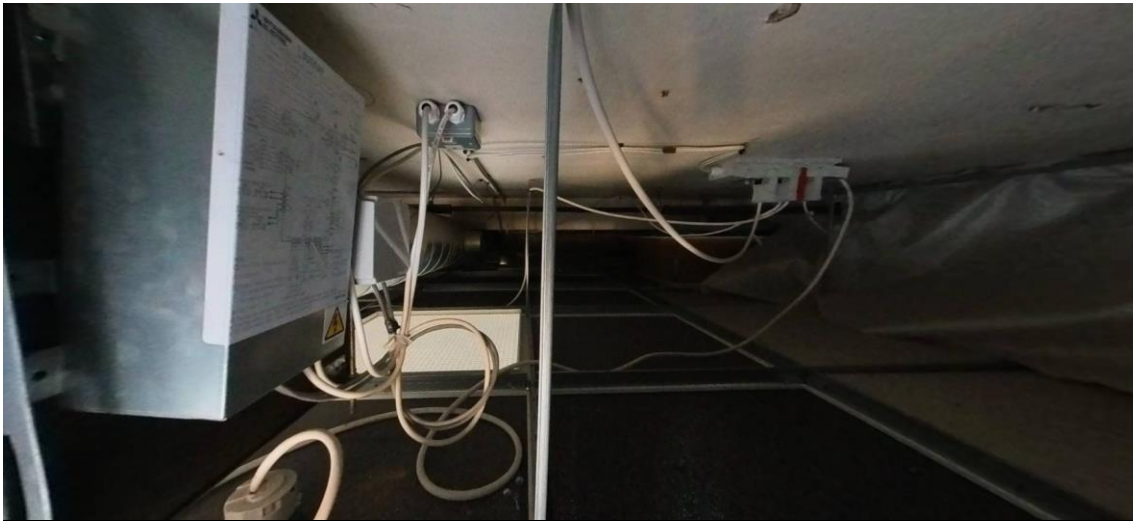
Plate 27: Above suspended ceiling line.
