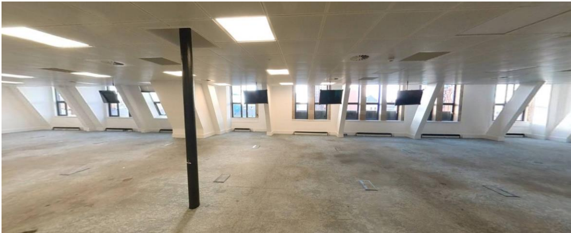
Plate 9: Main office space
