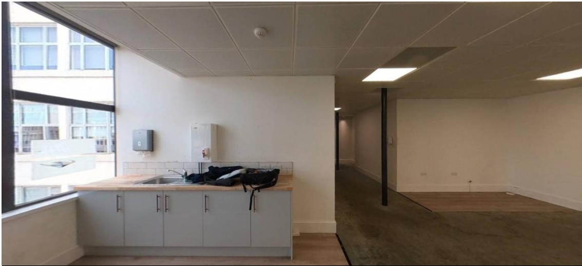
Plate 3: Main office space. Existing kitchen area.
