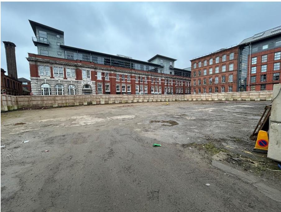
Figure 2: View across site in northern direction
