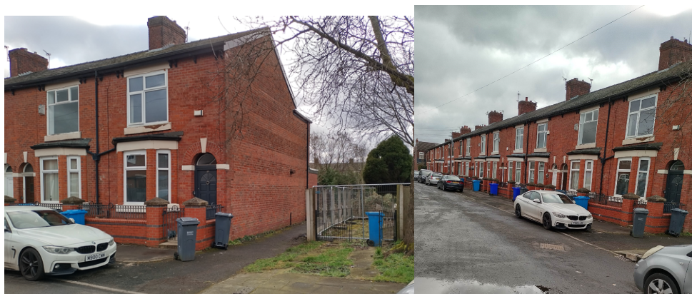
Fig.1 – Views of 29 Montana Square
