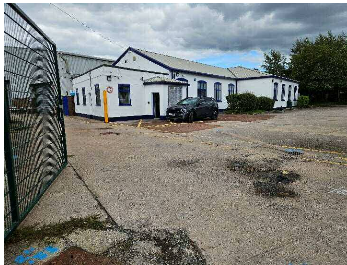
Photograph 2 – The office building in the south of the site. Viewed north.
