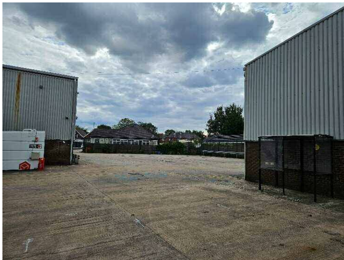
Photograph 5 – Present above ground fuel tank in left of image. Former above ground fuel tank in location of shelter.
