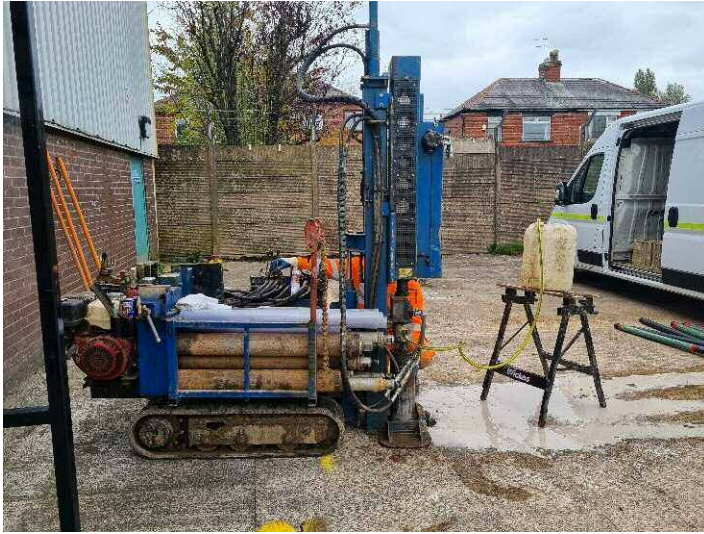
Photograph 9 – Location and drilling of borehole WS01.
