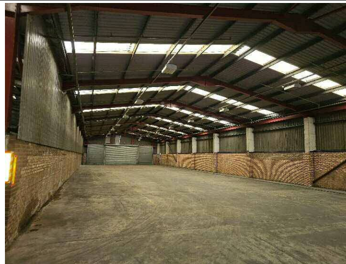
Photograph 8 – The northern warehouse.
