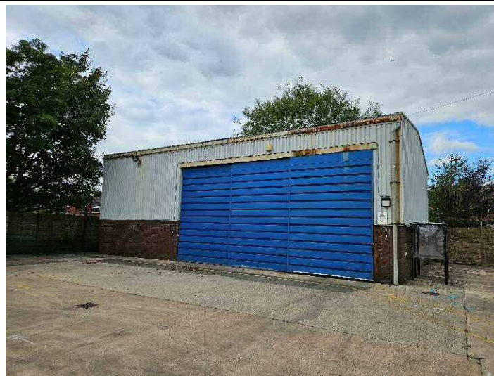
Photograph 4 – Former vehicle maintenance building.
