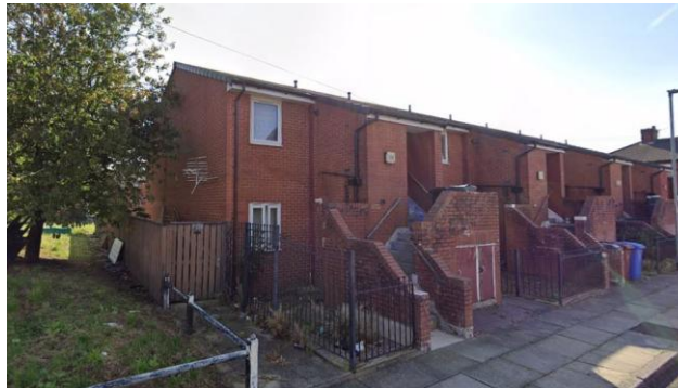
View of the maisonettes located on Kennard Close and the side of the site.
