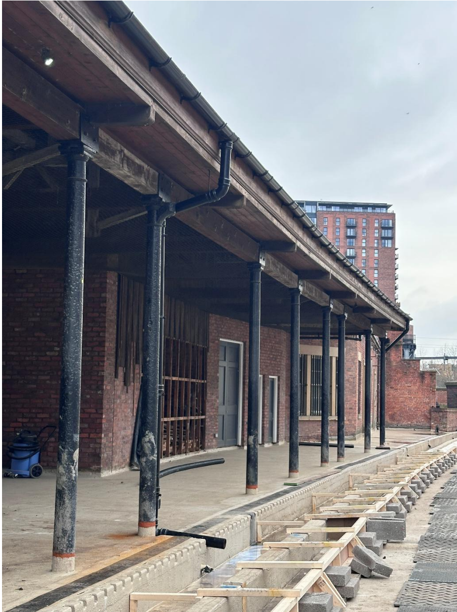
Photograph 7 – installed independent downpipe, concealed behind column to the west side
