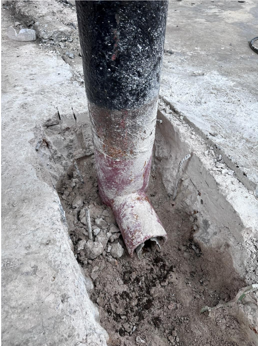
Photograph 5 – base of column with upvc lining pipe visible
