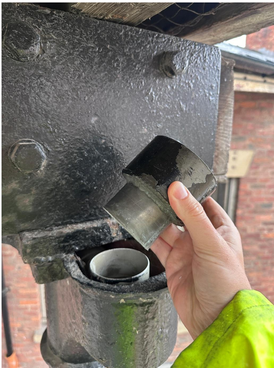
Photograph 4 – Head connection with internal column with removable lead spigot and upvc lining pipe visible
