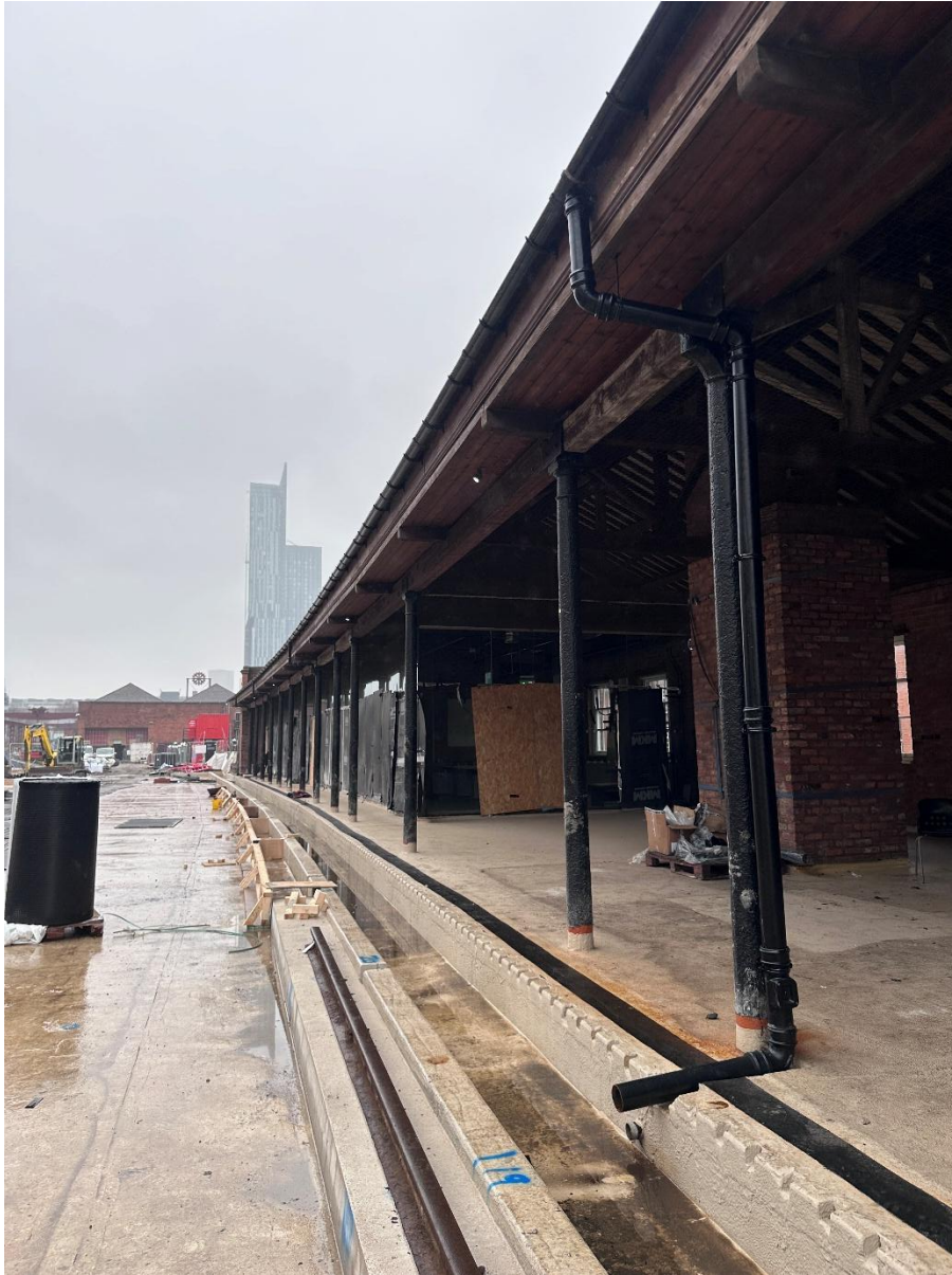
Photograph 9 – view from the west, looking east, showing new cast iron independent downpipe, dispersing into south trough
