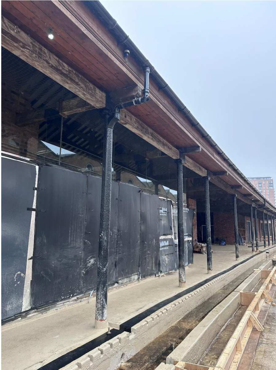
Photograph 6 – existing / current arrangement of transition pipe into internal lining pipe
