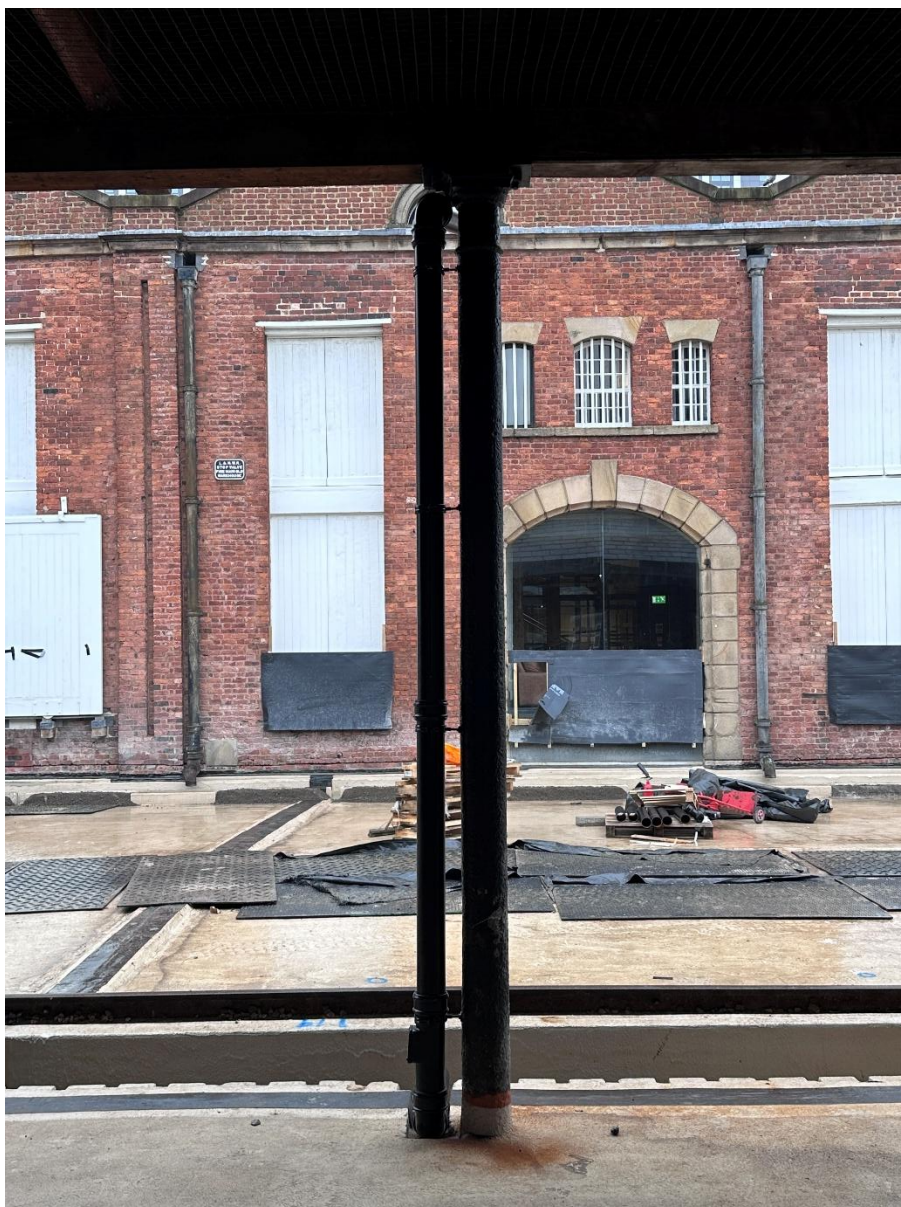
Photograph 8 – view from south within cover platform, showing new cast iron downpipe fixed into the side of existing column
