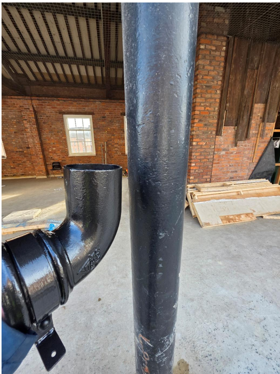
Photograph 11 – final sample of new cast iron downpipe including finish and bracketing
