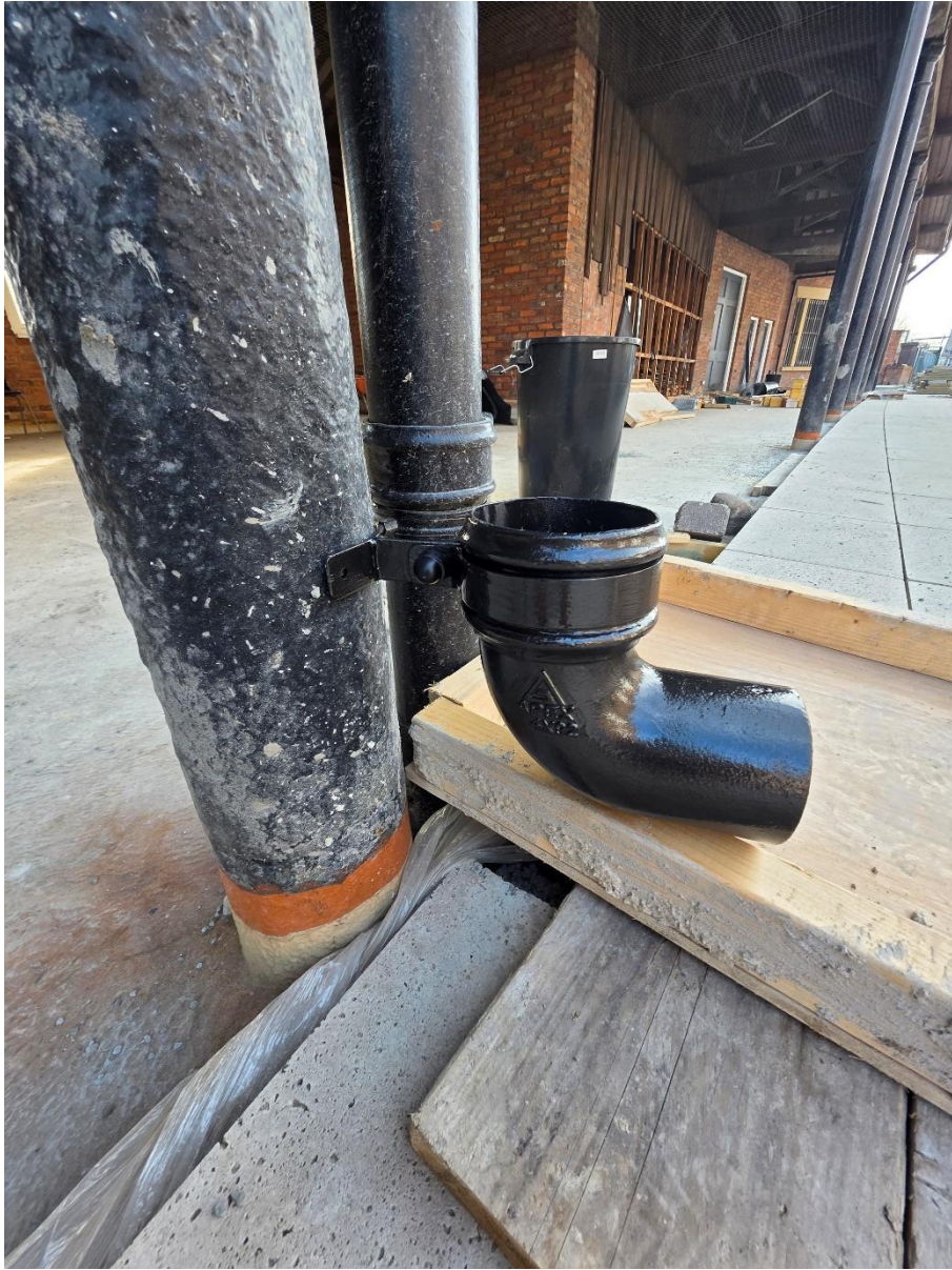
Photograph 10 – final sample of new cast iron downpipe including finish and bracketing
