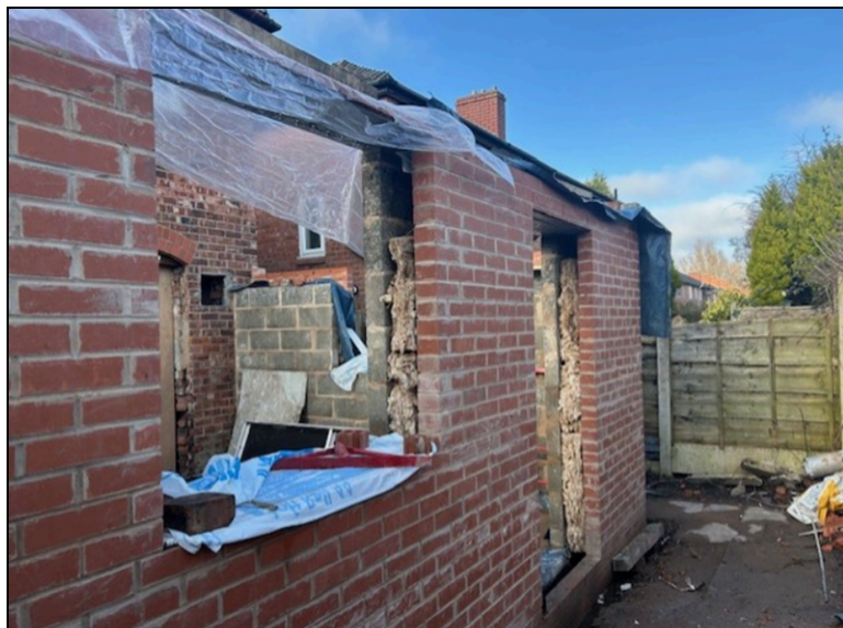
Rear extension under construction
