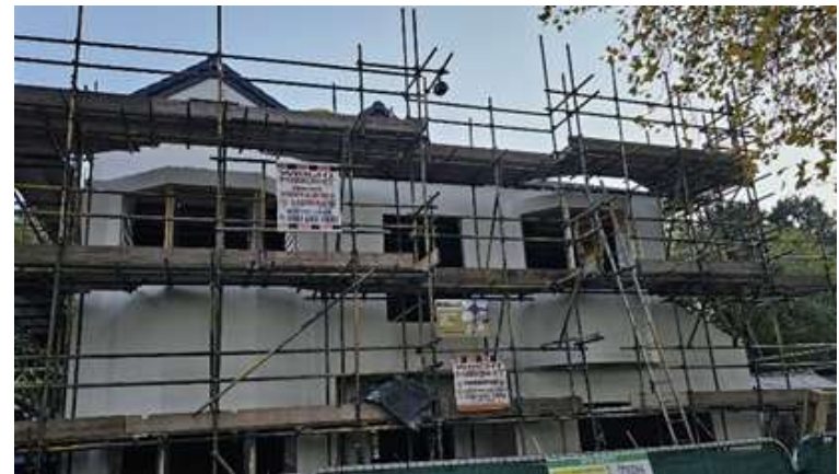
Image of construction of new dwelling
