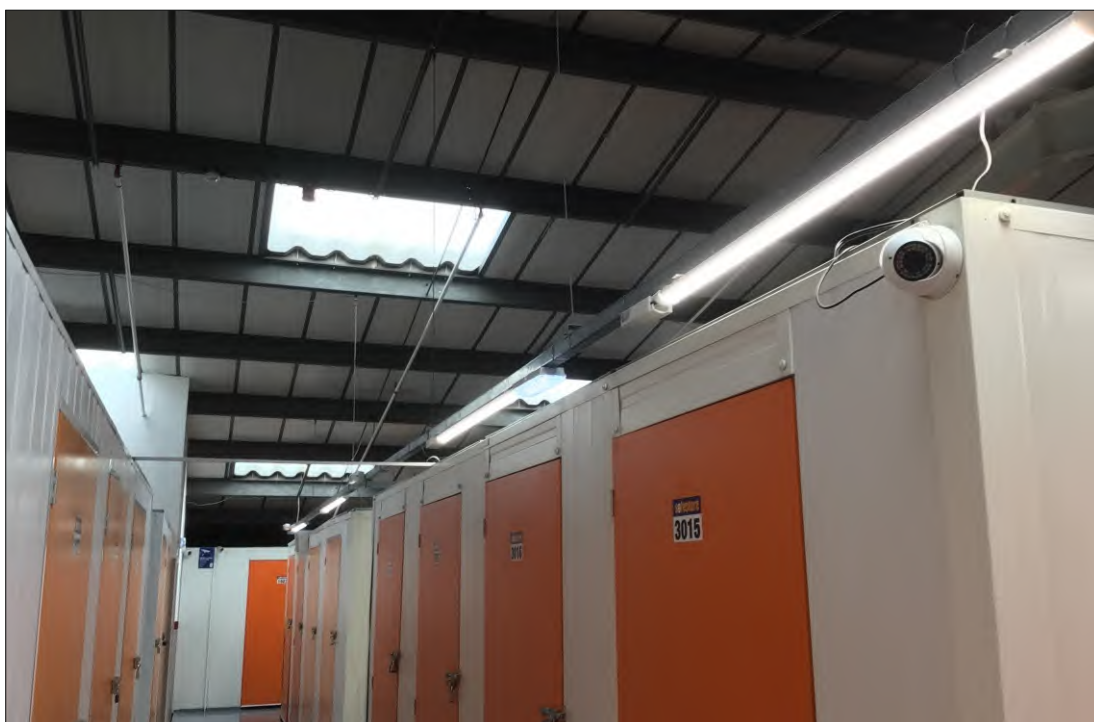
PHOTOGRAPH 2: Building B1 interior
