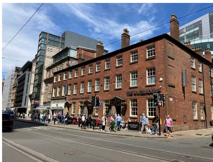
Figure 11: 65 Princess Street- June 2022
