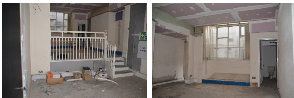
Interior photos looking towards the rear of the existing open space including 'art-deco' bay window to become new back bar display
