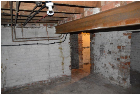
Front basement store area
