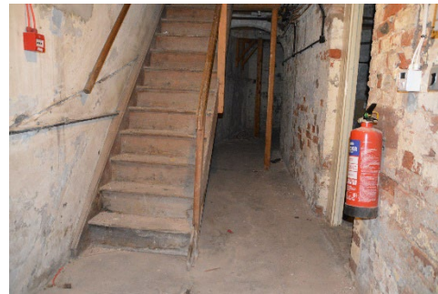
Existing staircase to basement
