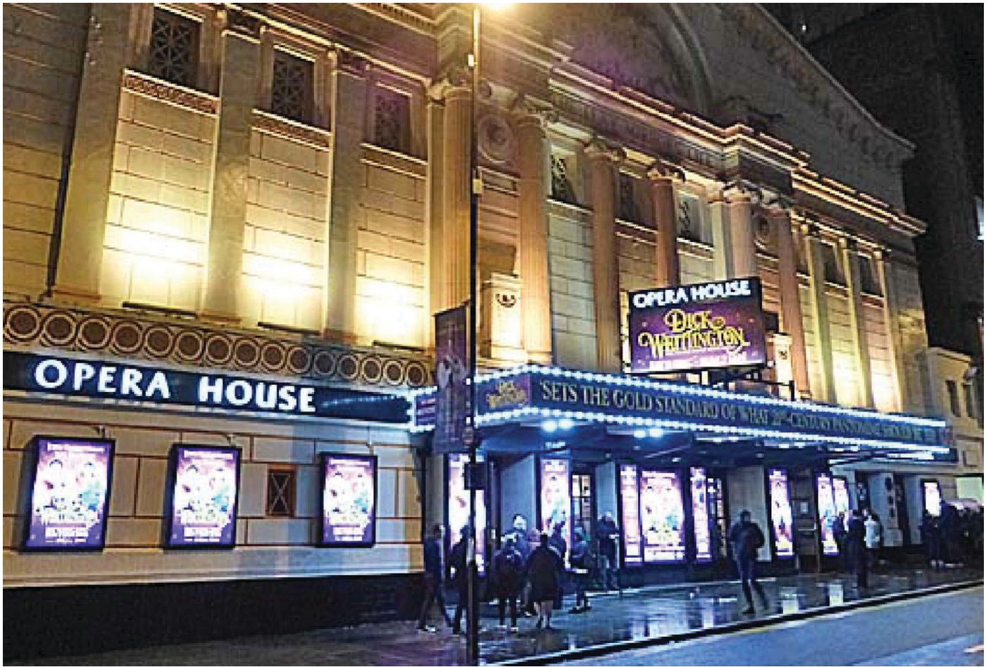
Existing illuminated signage.
