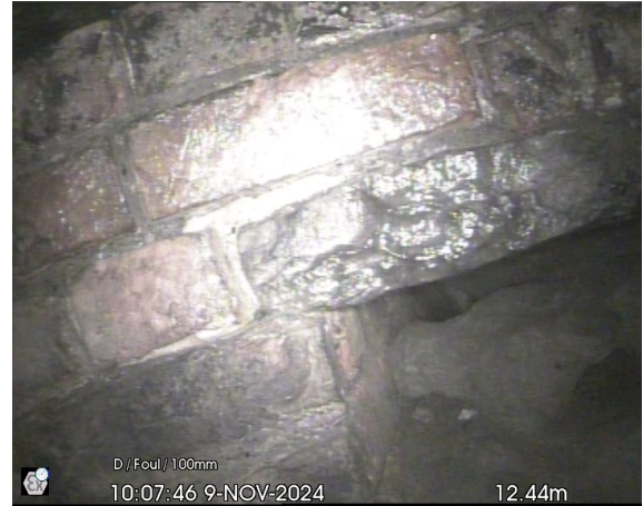
UU3FW-MAIN_12-44m_100746.jpg, 00:01:00, 12.44 m Finish node type, outfall, reference number: MAIN
