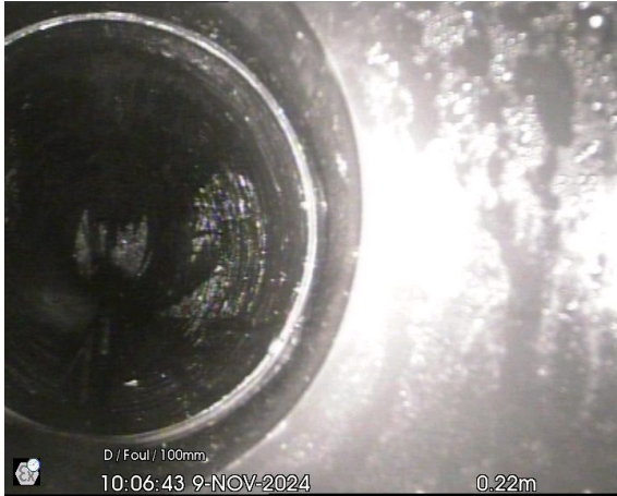
UU3FW-MAIN_0-22m_100643.jpg, 00:00:11, 0.22 m Junction, at 03 o'clock, diameter: 100 mm
