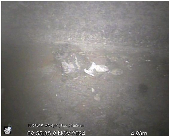
UU2FW-MAIN_4-93m_095535.jpg, 00:00:38, 4.93 m Finish node type, outfall, reference number: MAIN
