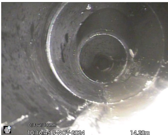
UU4FW-MAIN_14-20m_101645.jpg, 00:01:02, 14.20 m Junction, at 12 o'clock, diameter: 100 mm
