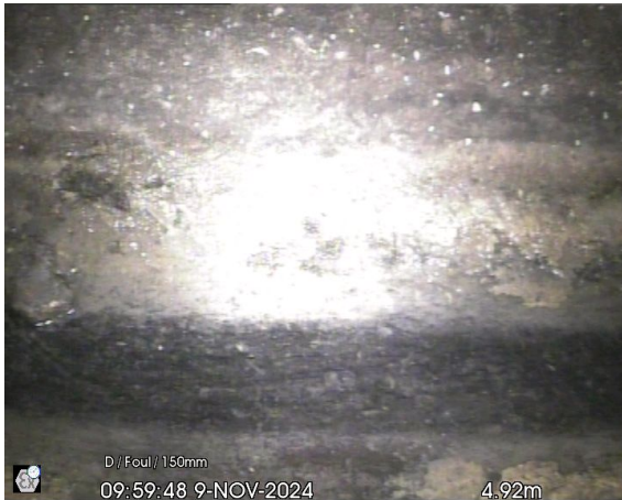
UU1FW-MAIN_4-92m_095948.jpg, 00:00:41, 4.92 m Finish node type, outfall, reference number: MAIN
