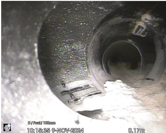
UU4FW-MAIN_0-17m_101535.jpg, 00:00:07, 0.17 m Junction, at 09 o'clock, diameter: 100 mm
