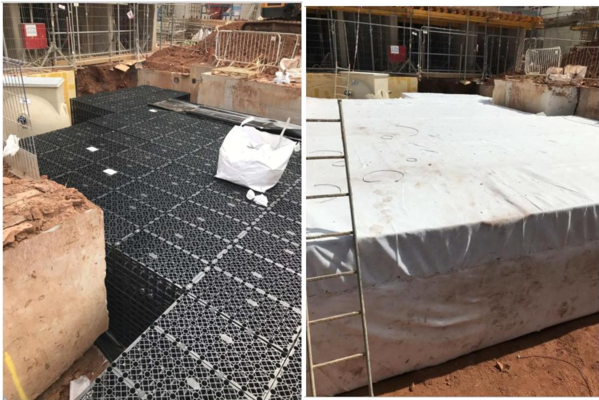
Figure 1 – Attenuation tank installation
