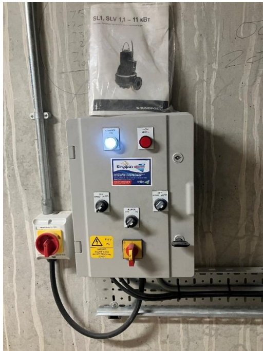
Figure 2 – Pumping Station installation
