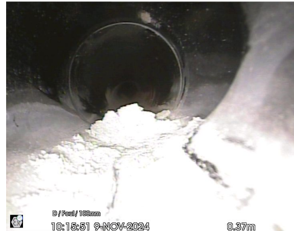
UU4FW-MAIN_0-37m_101551.jpg, 00:00:17, 0.37 m Junction, at 03 o'clock, diameter: 100 mm
