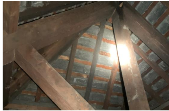
Picture 14 – Well sealed internals of R1
