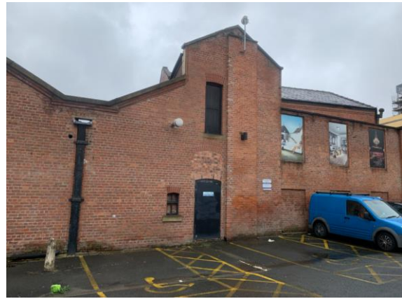
Picture 4 – Eastern aspect & pitched roof
