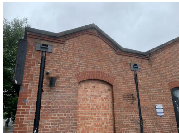
Picture 6 – Southeastern corner aspect
