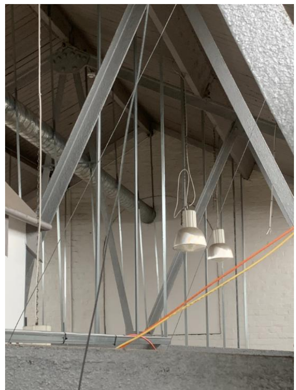
Picture 18 – Northern warehouse roof space
