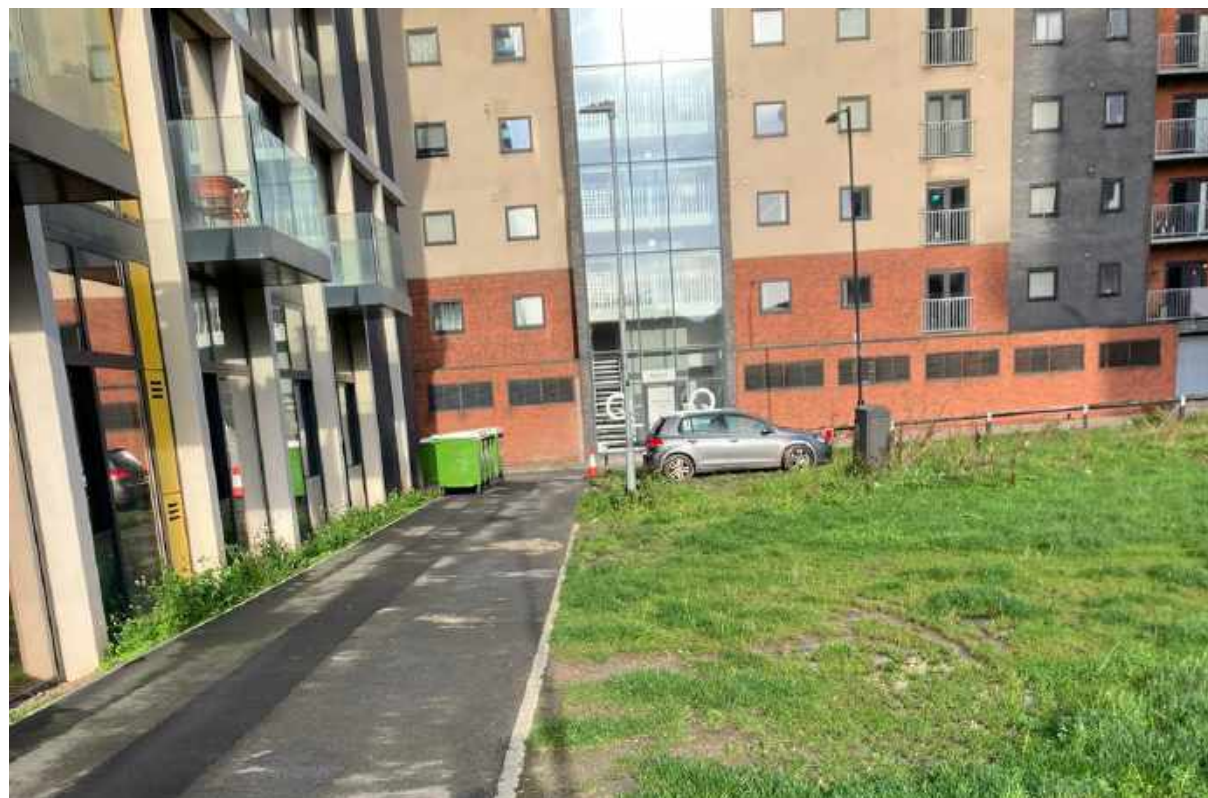
Photograph 2 – Looking along the pathway and apartment building on the western boundary.
