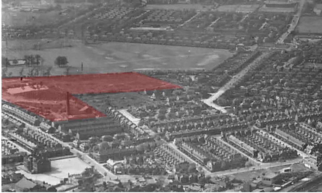
Figure 11: 1949 aerial photograph looking north-west across the Site (approximately shaded red) which had been owned by J&A Jacksons Ltd for 22 years at this time. (Source: Historic England)
