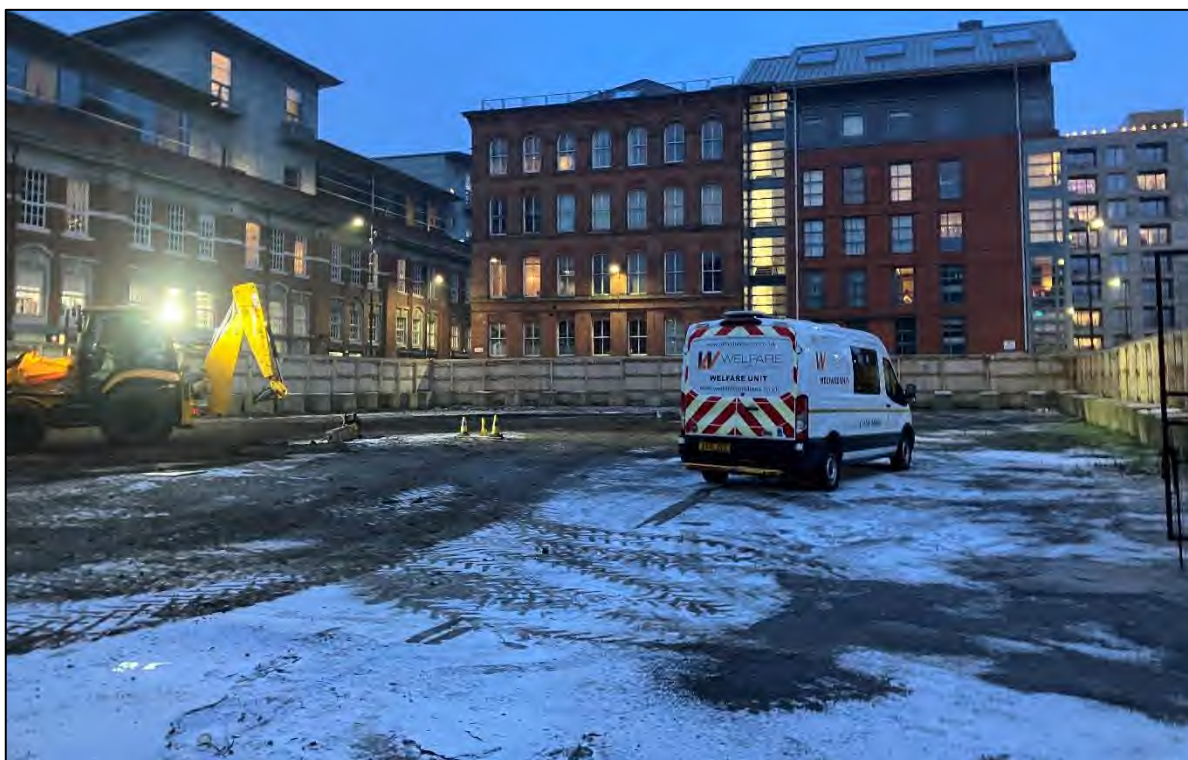
Figure 2-B: General view of the site, taken adjacent to the site entrance in the southeast facing north
