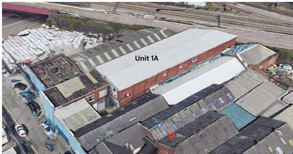
Figure 2.1 – View of Unit 1a looking North East
