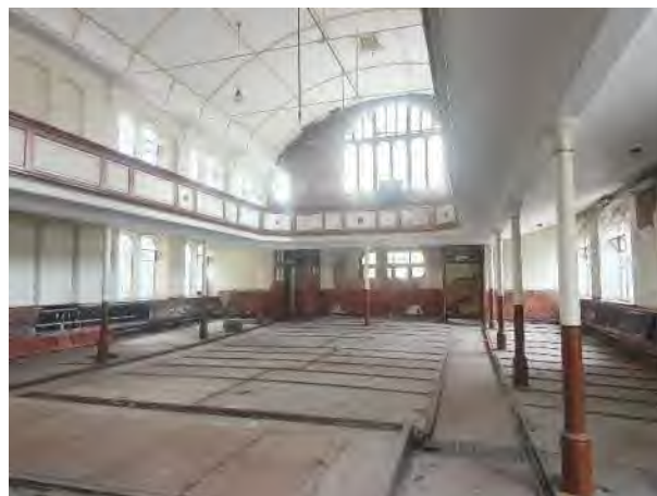
10. Ground floor of church hall.
