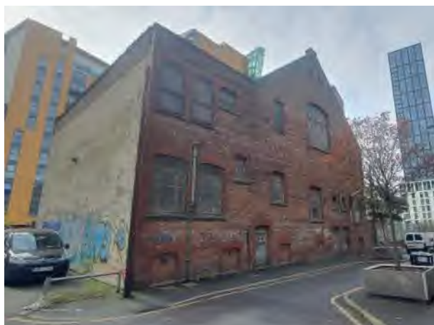
3. Northeast of site (looking southwest)
