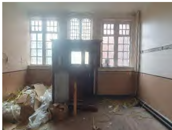
8. Ground floor side entrance (see picture 5 for external)
