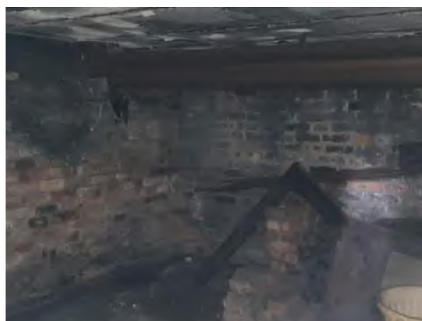
6. Basement void beneath the northeast of the church
