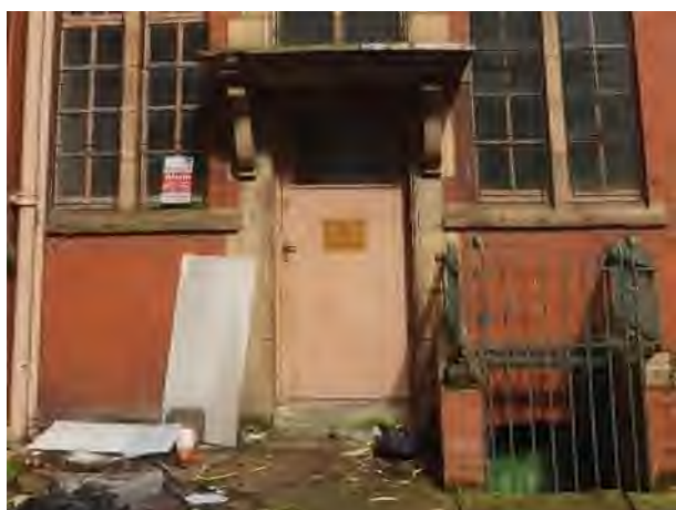
5. Basement access (down) and side access to church
