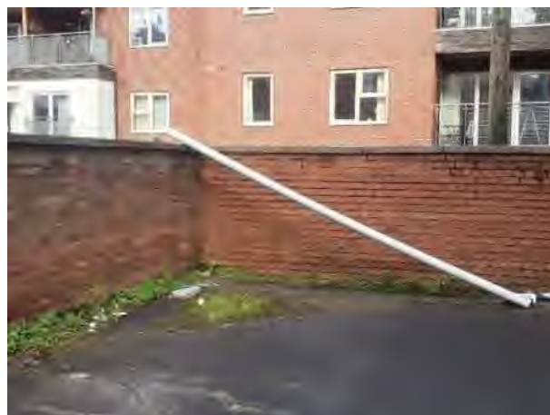
4. Concrete paving west of church
