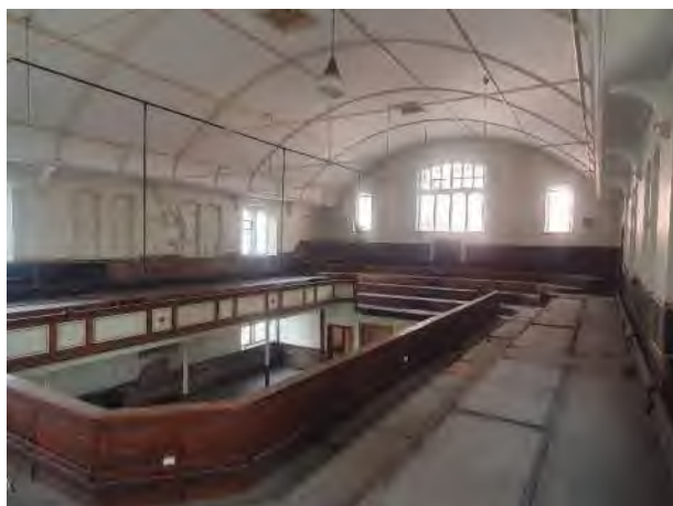
11. Mezzanine floor of church hall.
