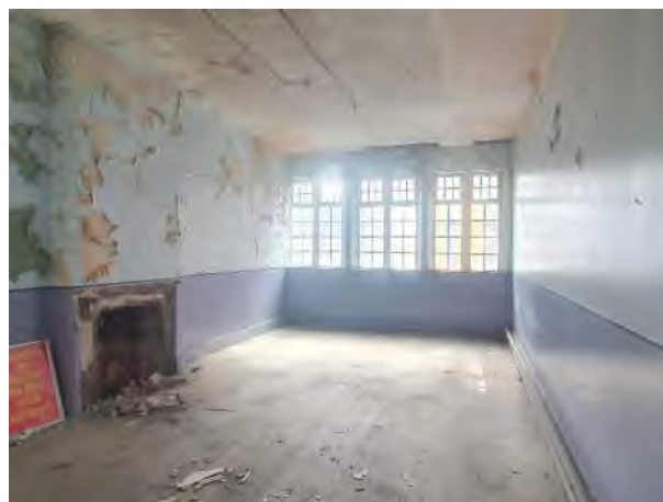
12. Mezzanine dining room.
