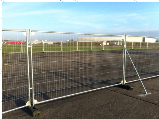
Heras tree protection fencing
