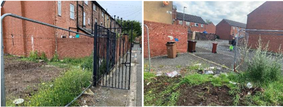
Figure 5: Photographs showing the northwestern corner of the site (left) and the site access looking north towards Milne Close (right).
