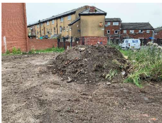
Figure 9 – Looking north west across the site.
