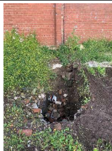
Figure 12 – Open hole in the western site section.
