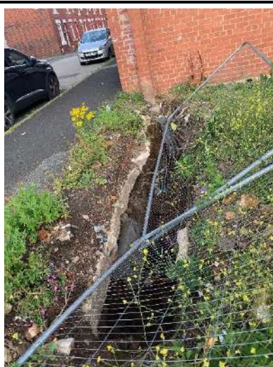
Figure 11 – Open hole running along the southern boundary.
