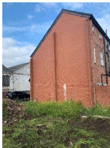
Figure 8 – Showing the hieght of the third party walls along the western boundary.
