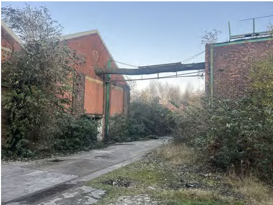
Figure 3: A view of self-seeded trees around dilapidated buildings.
