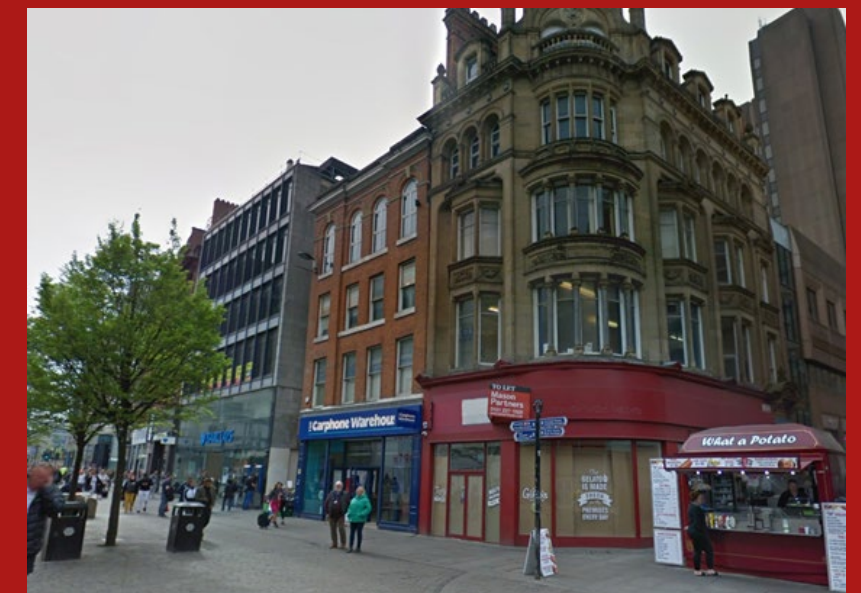
View of existing building seen from Market Street
