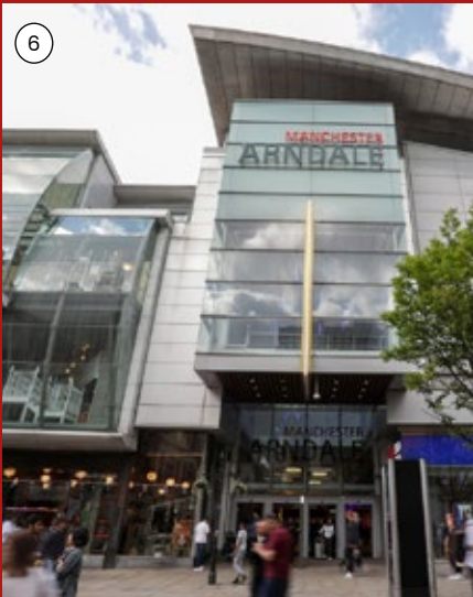
Arndale shopping centre - market street entrance
