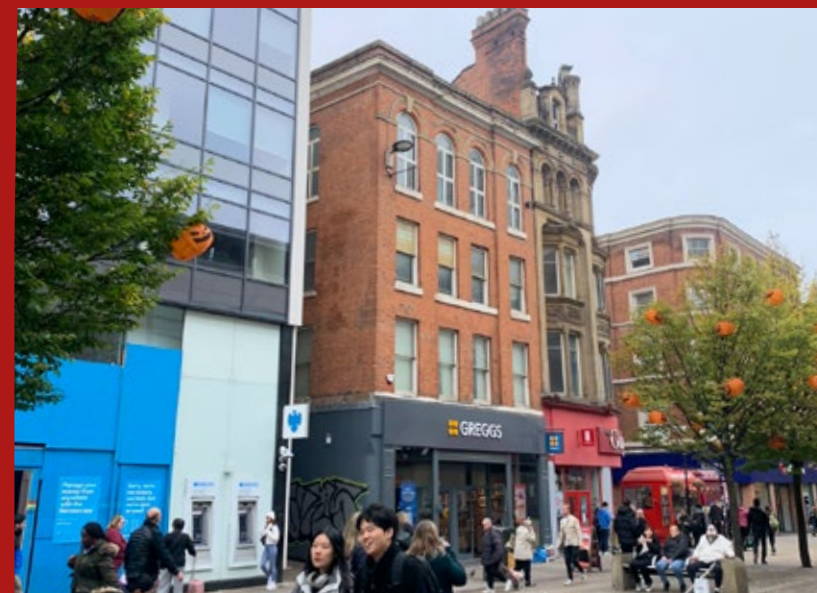
View of existing building seen from Market Street
