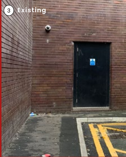
Existing security measure includes a security camera near the proposed entrance to apartments
