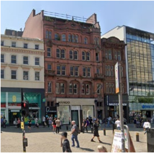
Traditional red brick building, 90-100 Market St.
