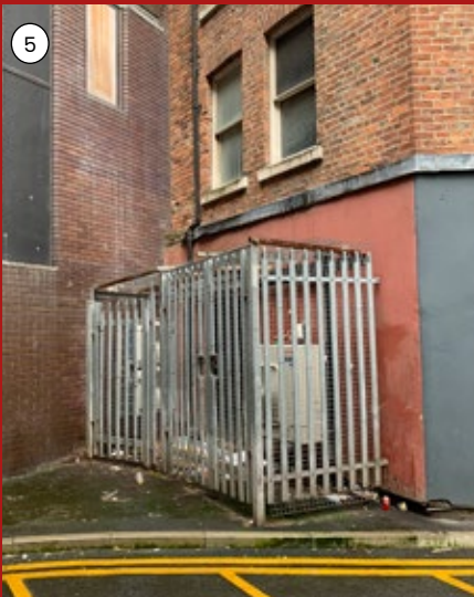
Rear elevation where the entrance to the building is and where the proposed entrance porch will be
