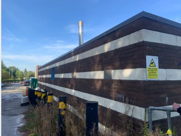
Photograph 9: A well-sealed building in the centre of the site
