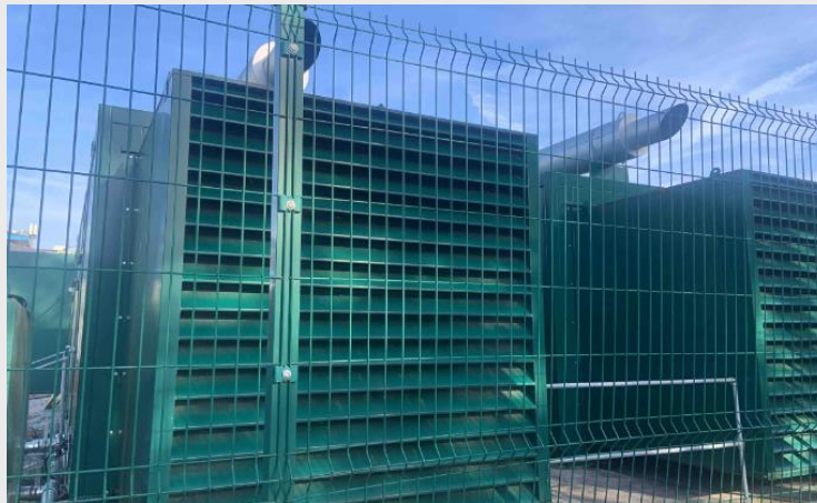
Photograph 8: Two ventilation structures within the centre of the site
