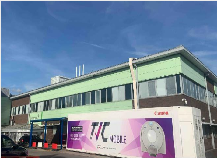
Photograph 3: Main building (B2) of the hospital
