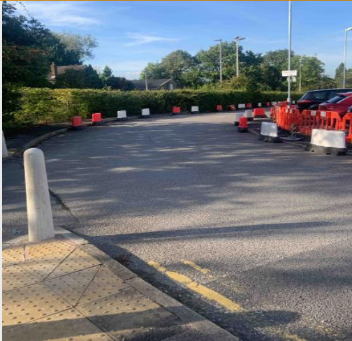
Photograph 1: Northern section of road into the carpark
