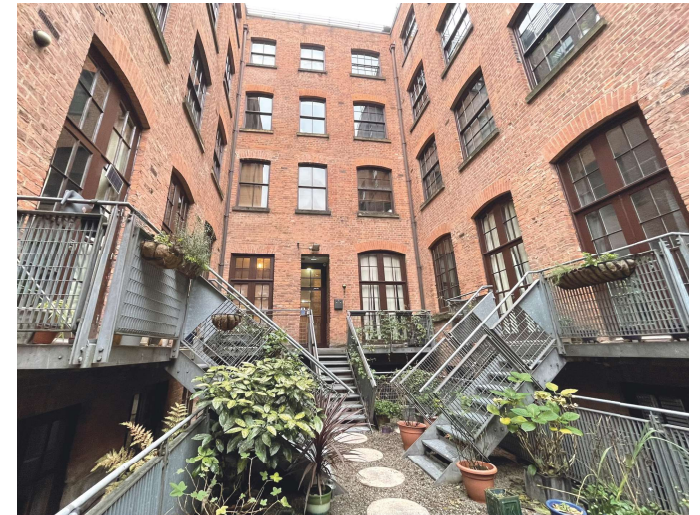
Fig. 03 Photo of rear courtyard facing St James Street
