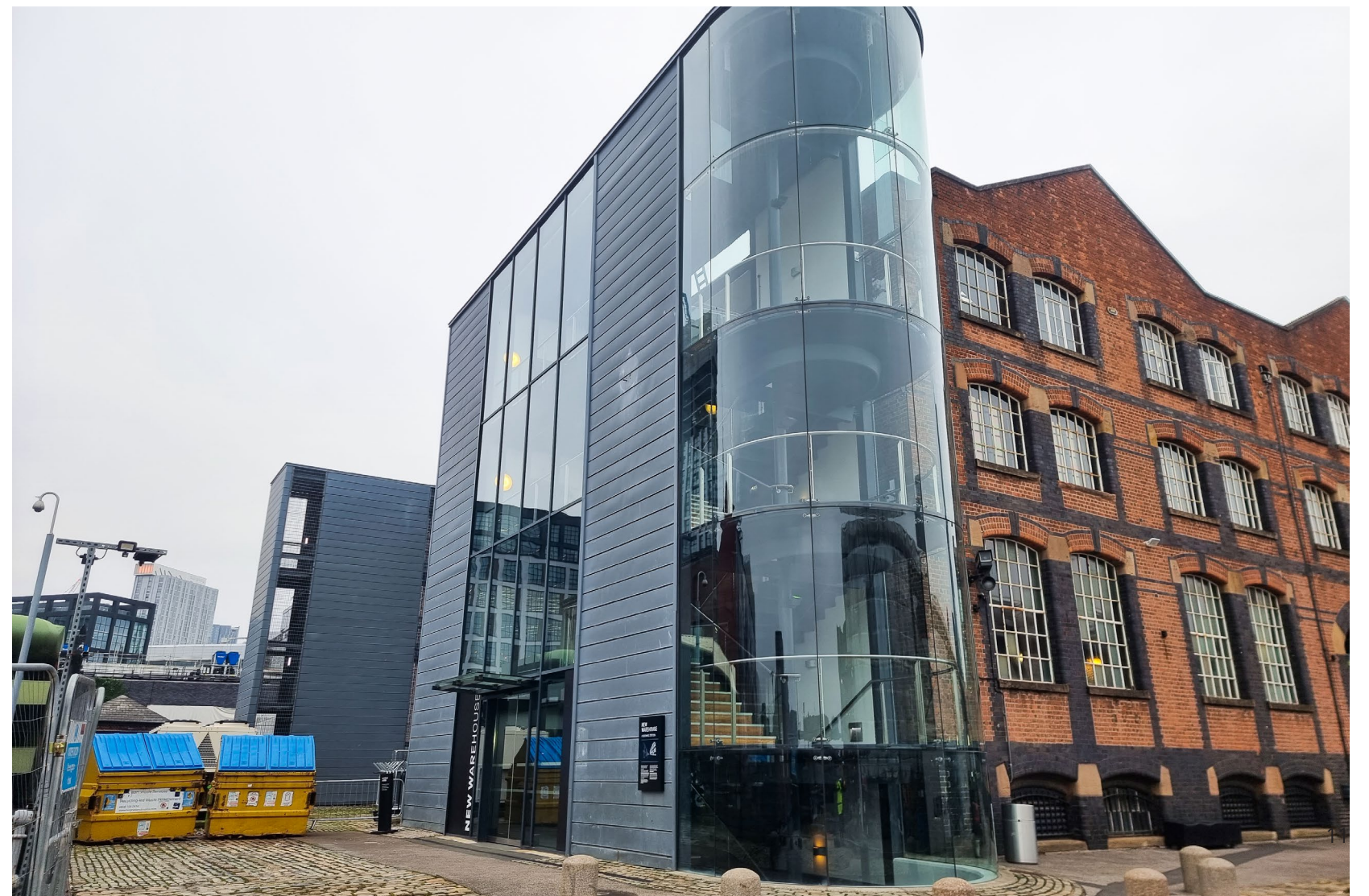
Figure 3 New Warehouse South Elevation and Upper Yard
