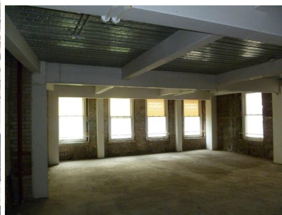
Figure 2.4 Second floor showing inserted steel frame encased in fire/sound insulation.
