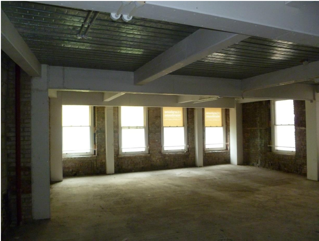
Second floor: no historic features aside from exposed brickwork.
