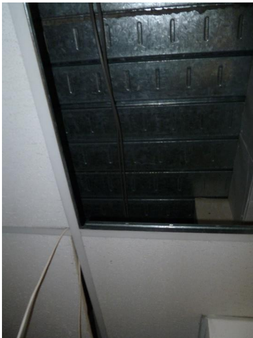
First floor: No historic ceilings above suspended ceiling.
