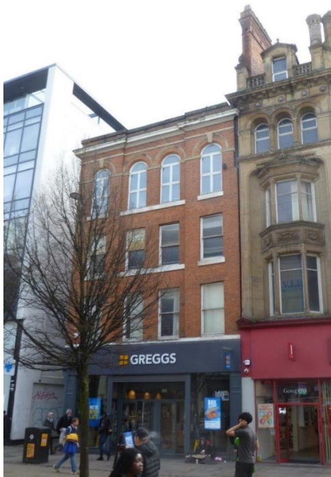
Figure 2.1: View of the building from Market Street.
