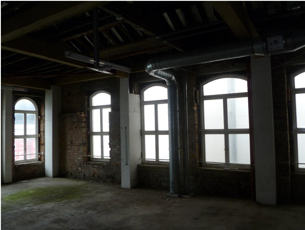
Third floor: Showing no ceilings or plasterwork are present.
