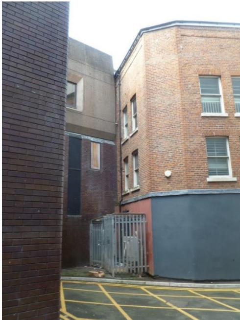
Figure 2.2: View of the rear elevation of the building from Sickle St showing the ground floor.
