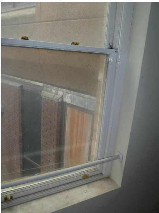
Windows throughout are modern timber frames with modern thin double glazed units.
