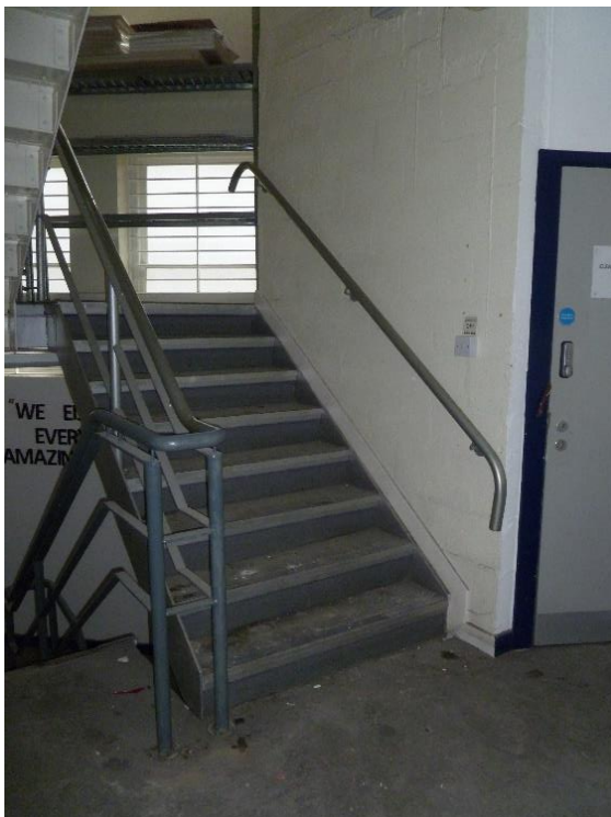
Inserted staircase leading to all floors.
