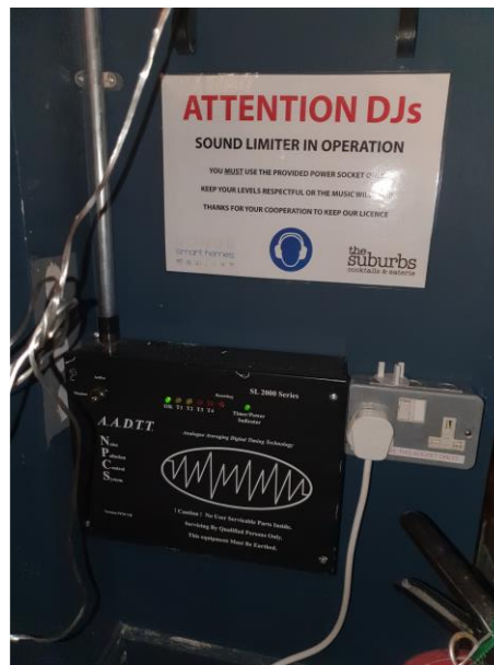
Figure 5 SL 2000 noise limiter
