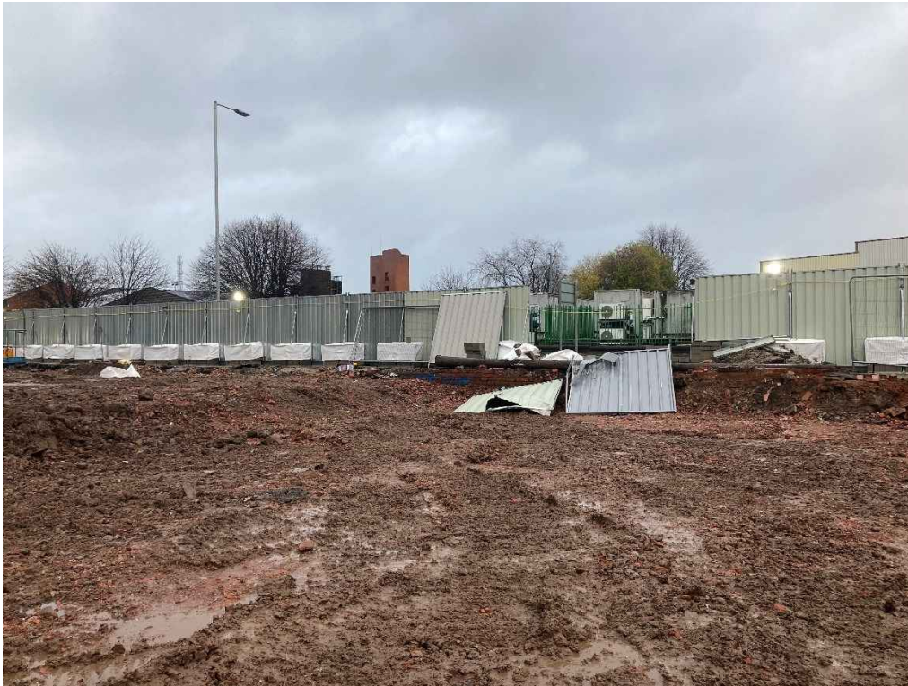
PLATE 11 VIEW OF SITE FACING EAST PRIOR TO PLACEMENT OF PILE MAT
