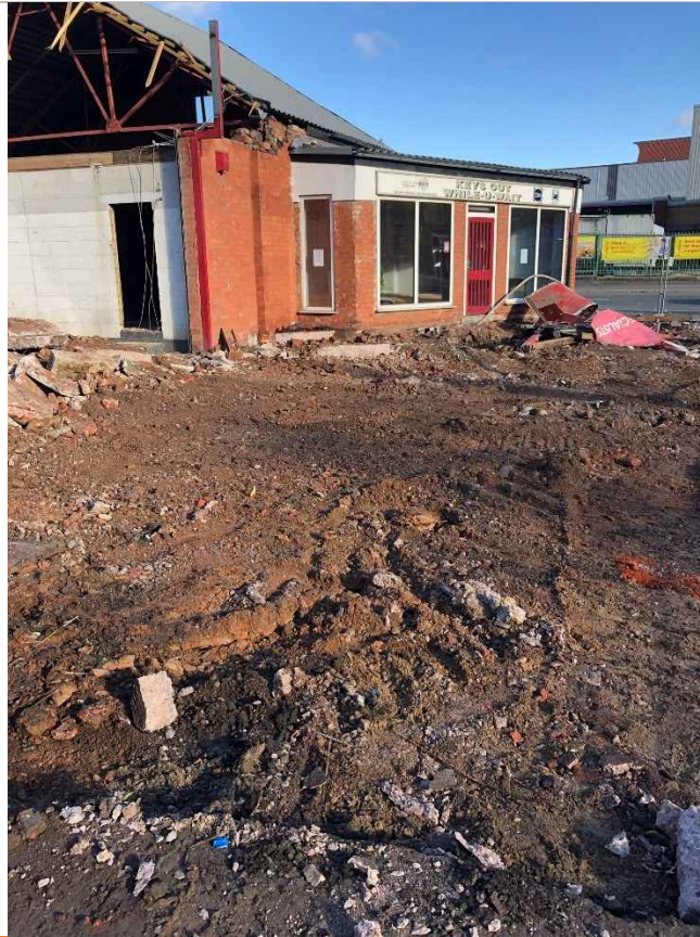
PLATE 2 EXCAVATION AND TURNOVER OF MADE GROUND
