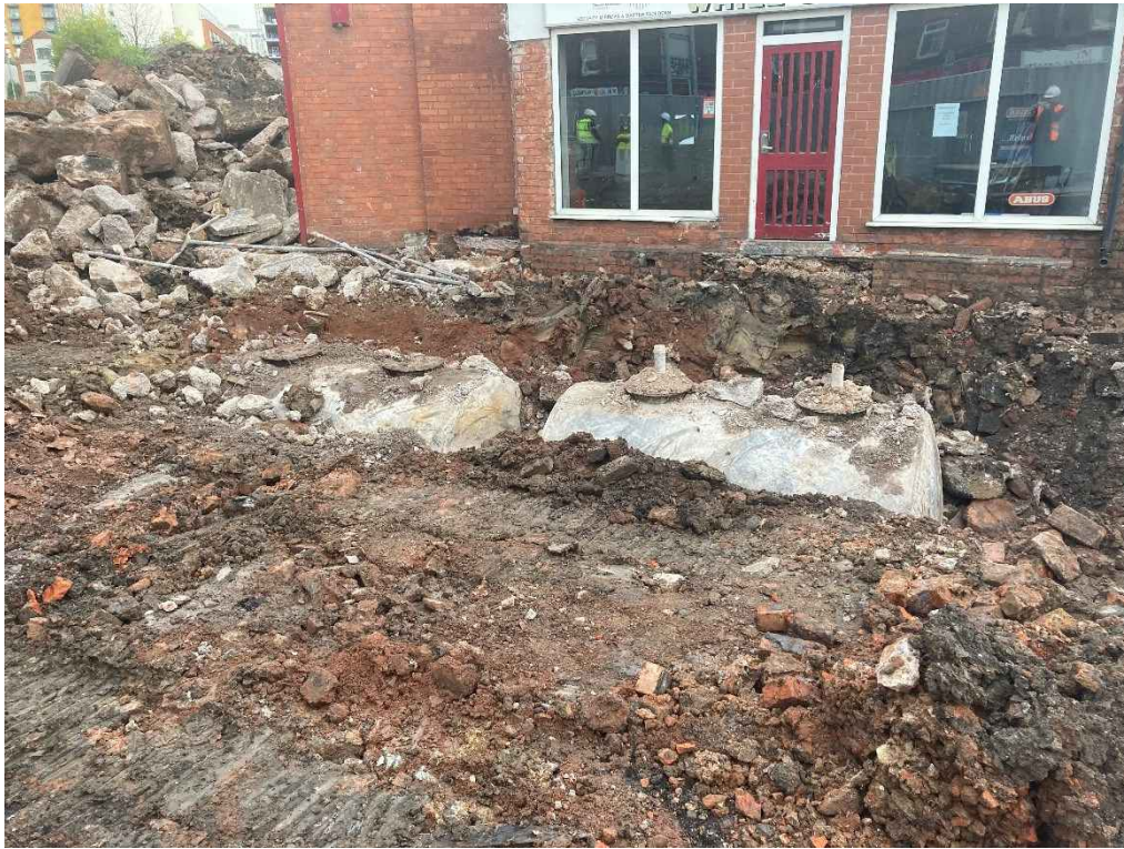
PLATE 3 EXCAVATION SURROUNDING TANK 1
