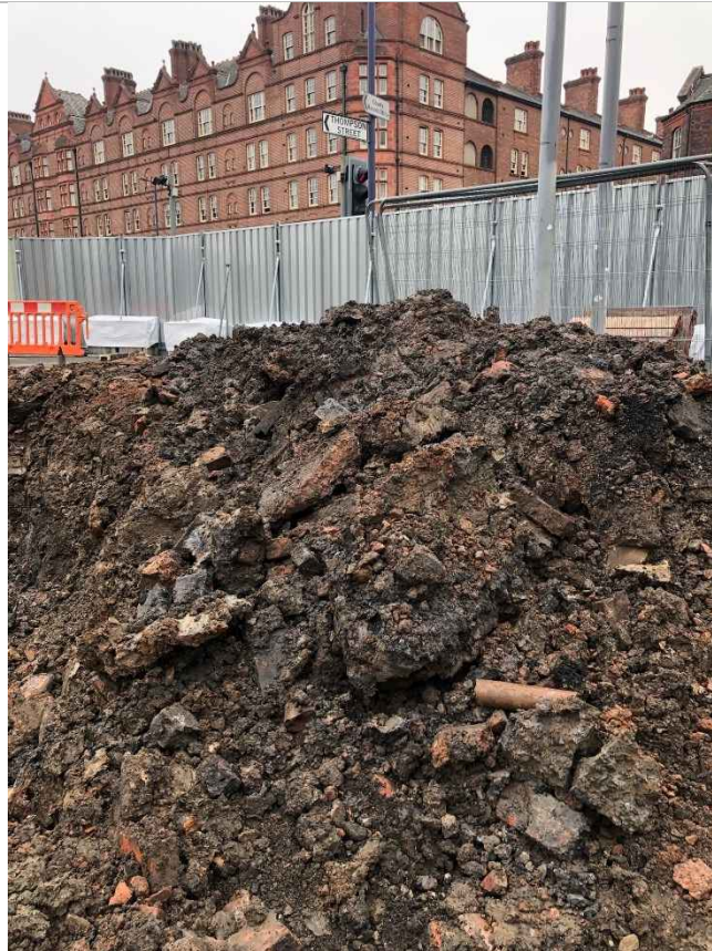
PLATE 9 ARISINGS FROM TANK EXCAVATION
