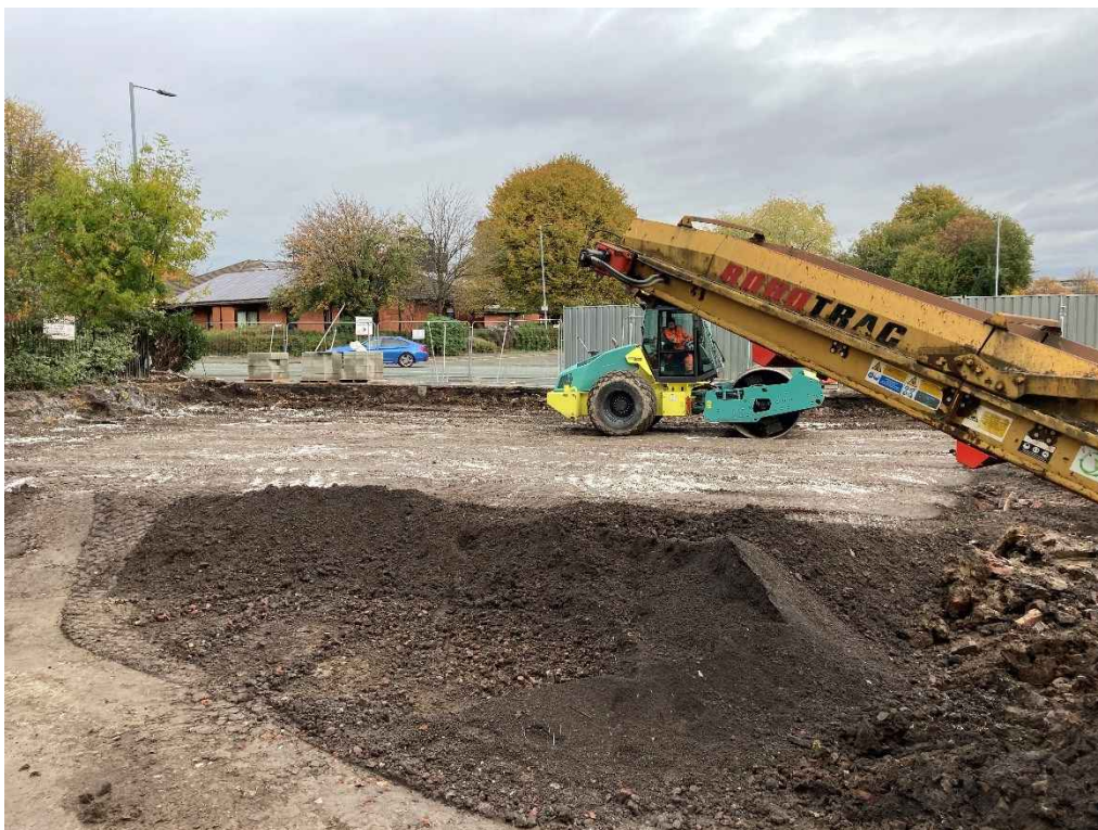
PLATE 12 VIEW OF SITE FACING NORTH – UNDERTAKING PLACEMENT OF PILE MAT
