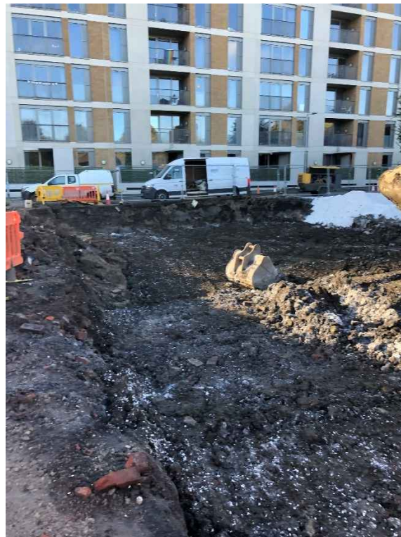
PLATE 2 EXCAVATION AND TURNOVER OF MADE GROUND
