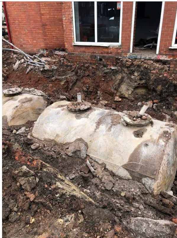
PLATE 4 TANK 1 IN SOUTH EAST OF SITE
