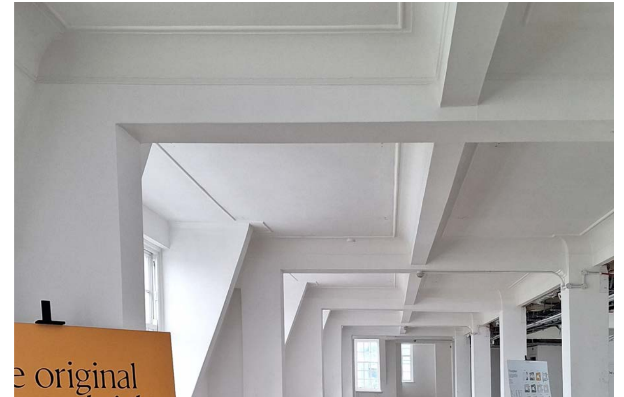
02 Existing coffered ceiling on Level 10
