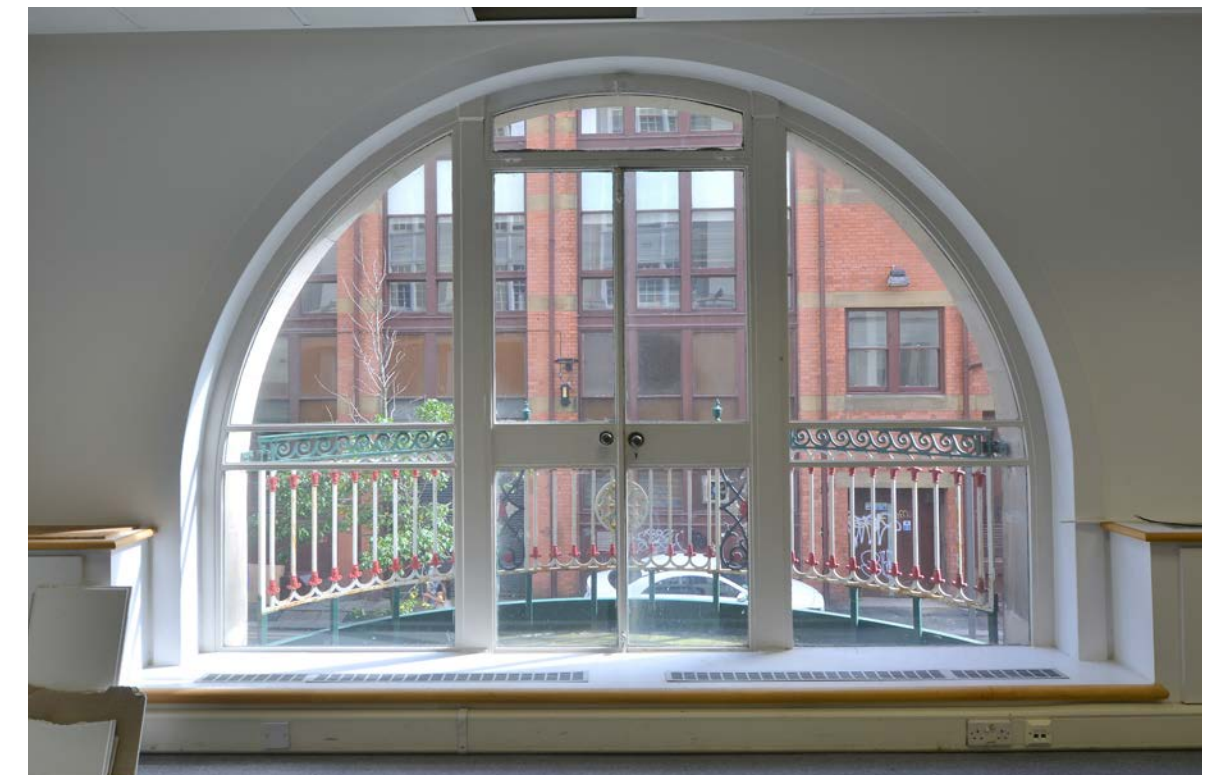
04 Arched window on Level 01
