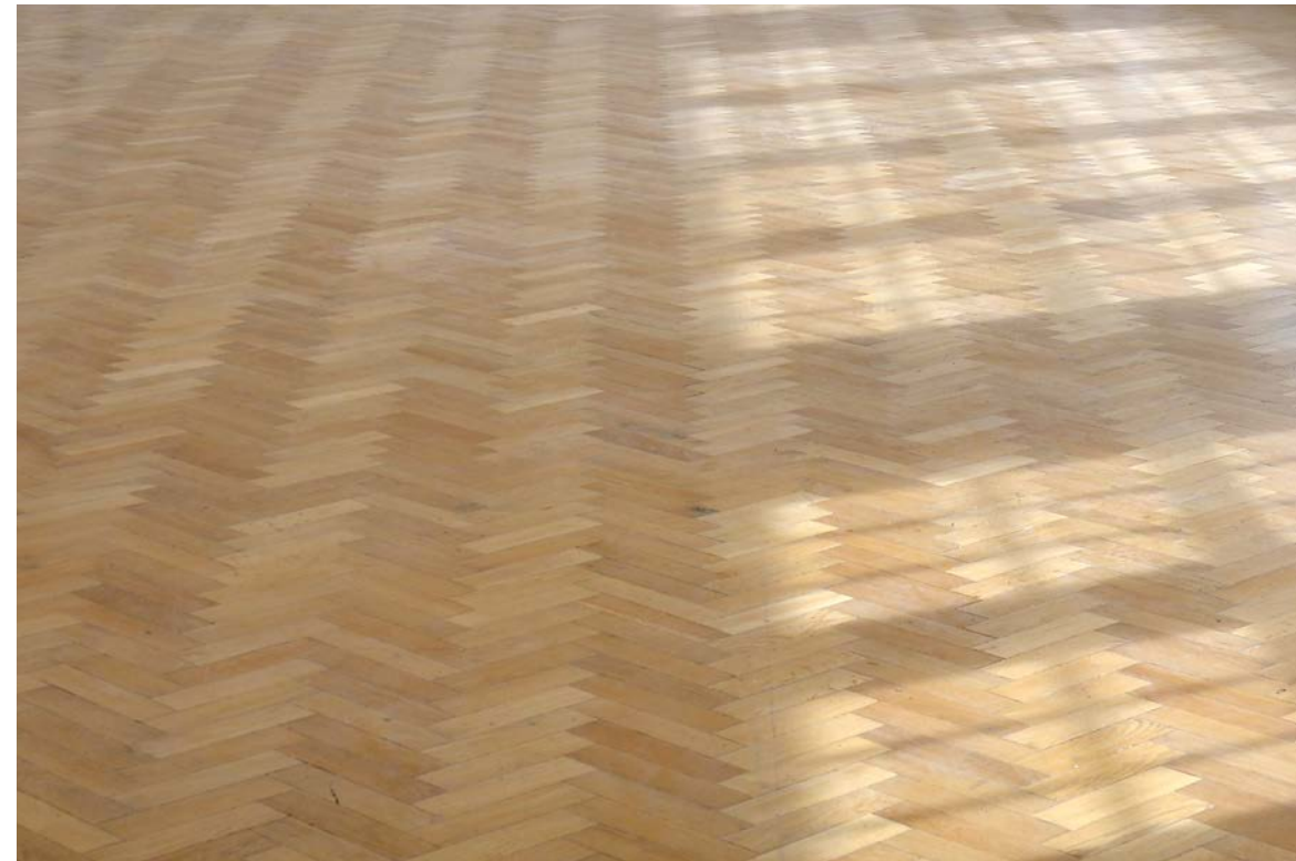
01 Existing parquet floor on Level 13
