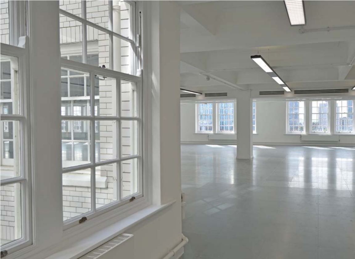
02 Internal sash windows
