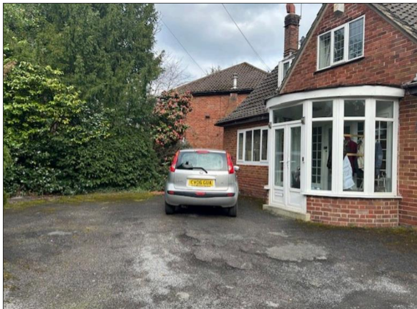
View of existing building
