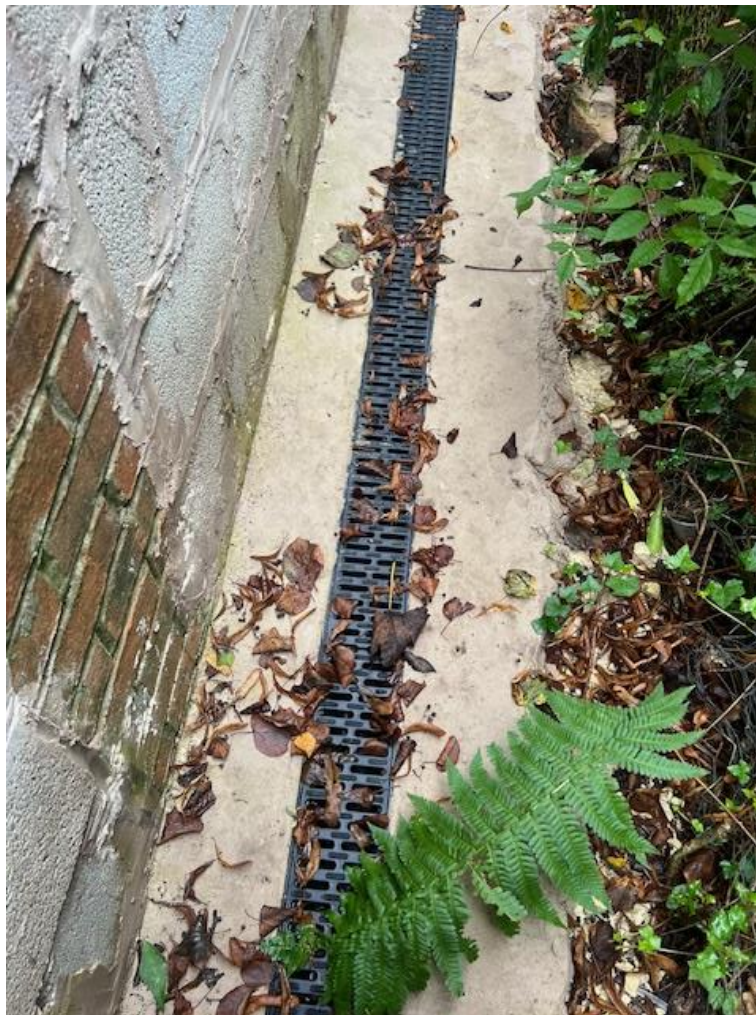
Drainage channels installed
