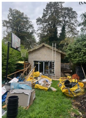
Partially constructed outbuilding
