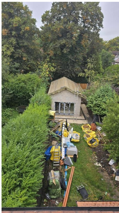
View of the partially constructed outbuilding from second floor rear elevation window – established vegetation to boundary with No. 26 Amherst to the left
