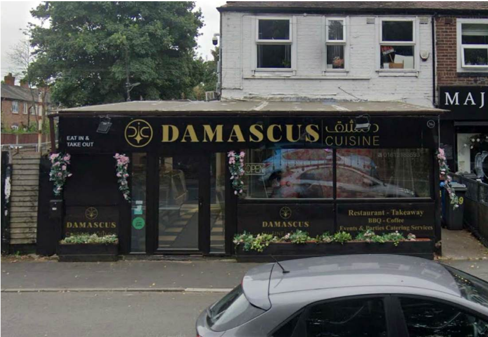
249 Barlow Moor Road (Damascus Cuisine) – A front extension approved under planning reference 108698/FO/2015/S1, which extends forward in a similar manner to the application site, reducing the visual impact of open forecourts. This structure remains in place, forming part of the area’s established character.
