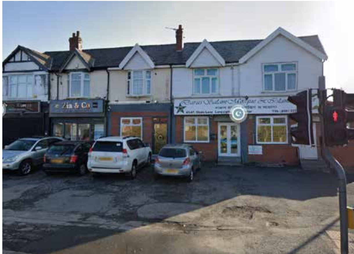
Front of existing building
