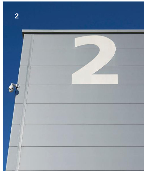
1: View of existing micro rib cladding in use at the Etihad Campus
