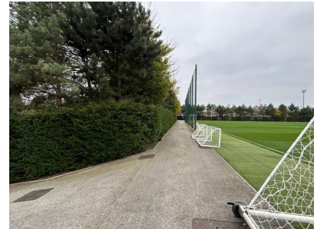
Below: View of the training pitches that are to receive underground heating and set at a higher site level than the site
