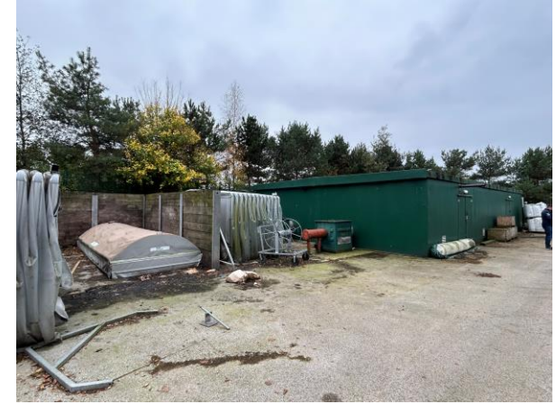
Above: View of the existing Filter House building on the south-West corner of the site and adjacent storage silos
