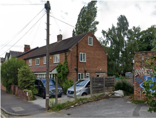
Existing building from the corner
