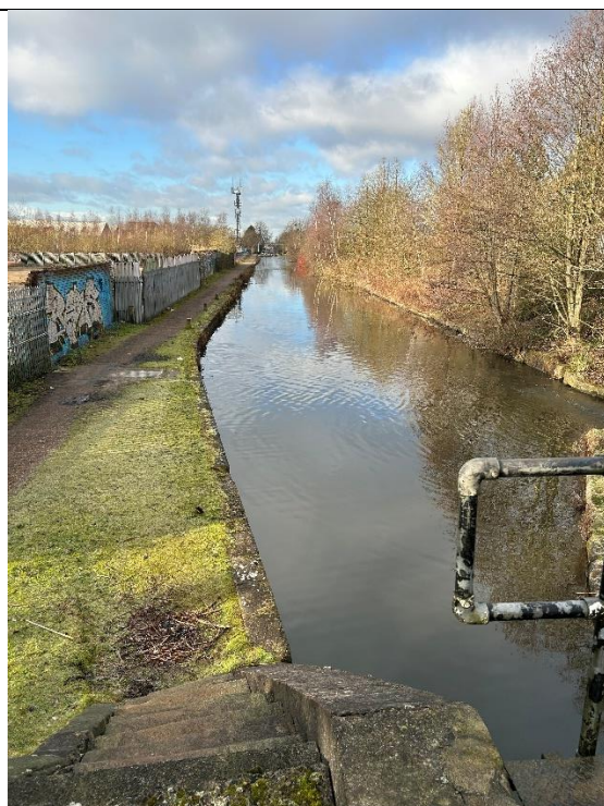
Photograph P05: View from Lock 14 looking west along Ashton Canal
