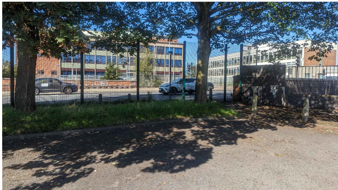
B1 - Ashton New Road, existing welded mesh fence boundary retained, vehicular gates removed & replaced with fencing panels to match existing
