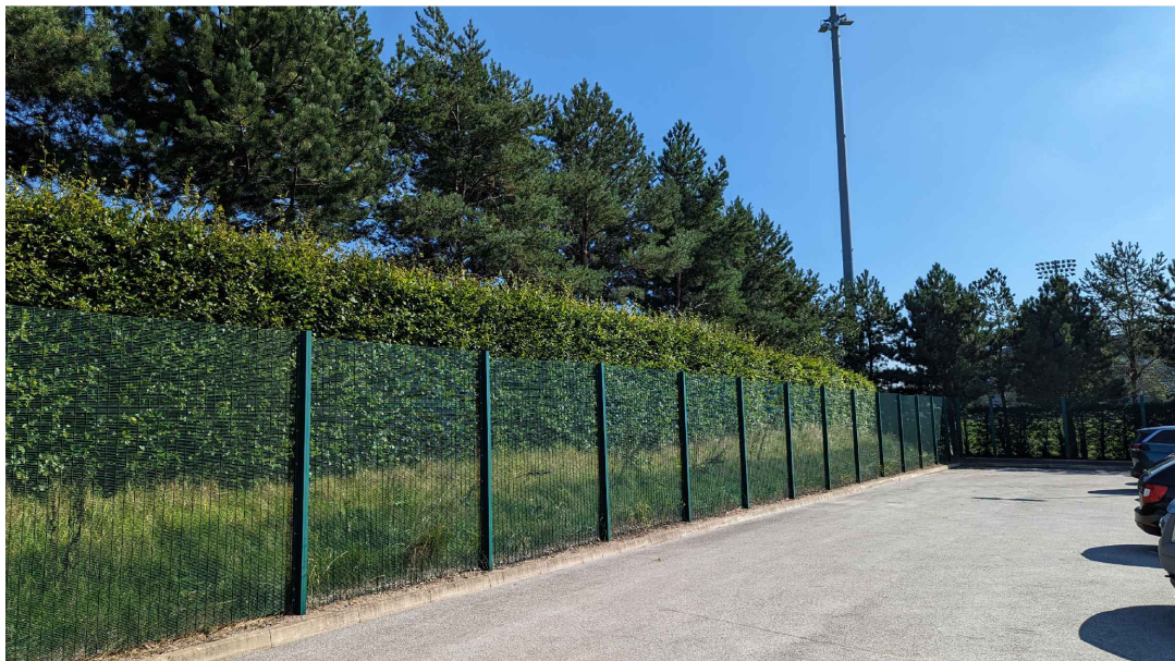
B4 - North car park existing welded mesh fence boundary relocated to new site entrance, new vehicular gates installed at site entrance
