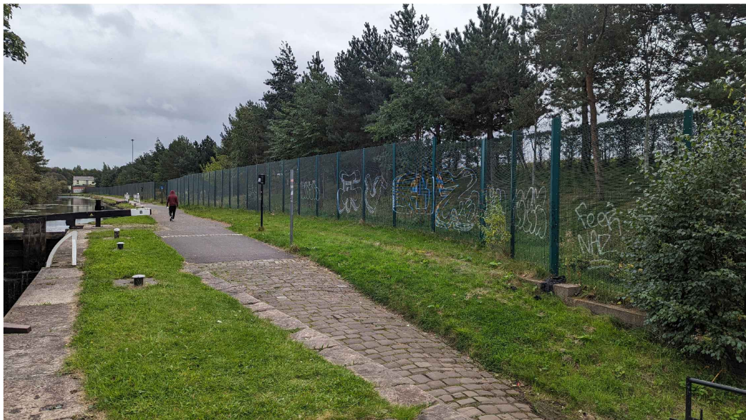
B3 - Surrounding welded mesh fence boundary retained
