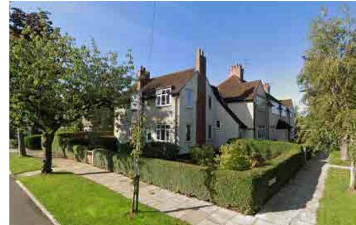
EAST AVENUE, BURNAGE GARDEN VILLAGE
