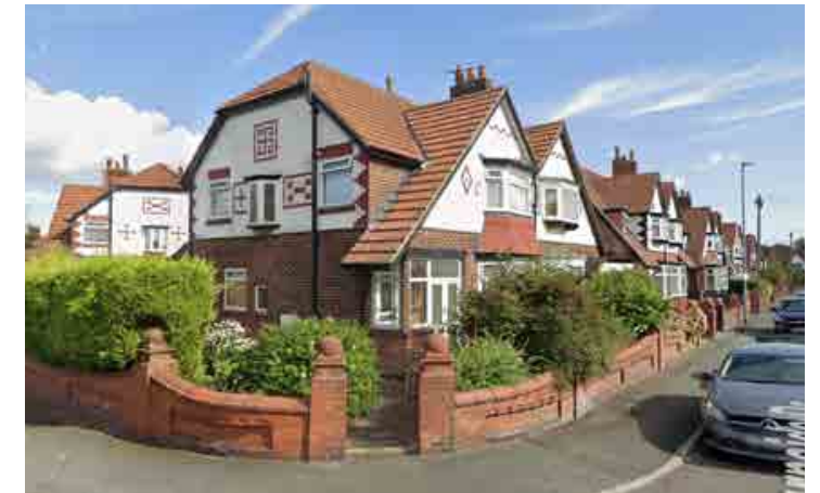
BURNSIDE DRIVE, NORTH OF SITE
