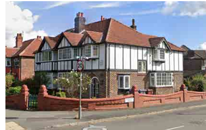
KINGSWAY, NORTH OF SITE
