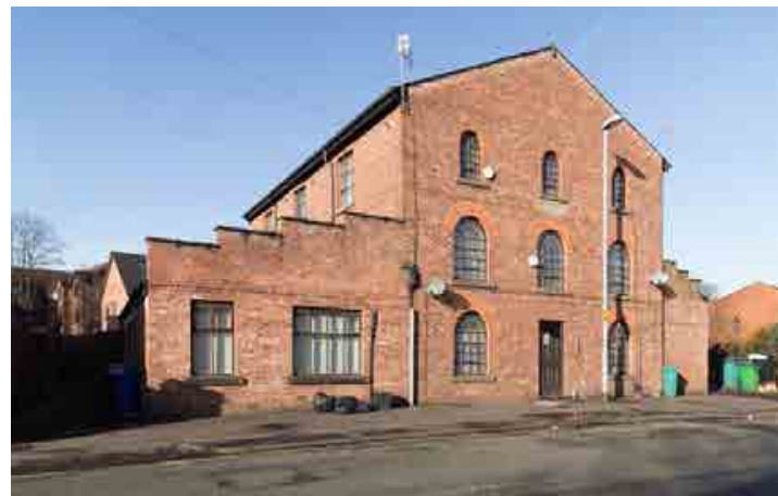
188, LADYBARN LANE, GRADE II
