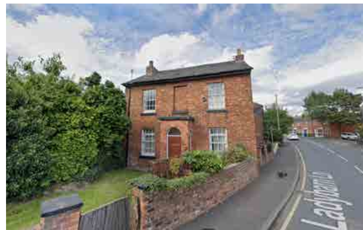
180, LADYBARN LANE, GRADE II
