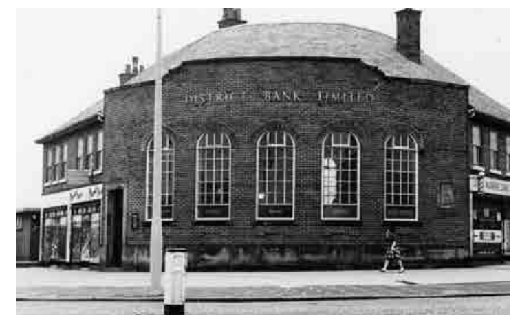
BURNAGE, MAULDETH ROAD/KINGSWAY, JUNCTION
