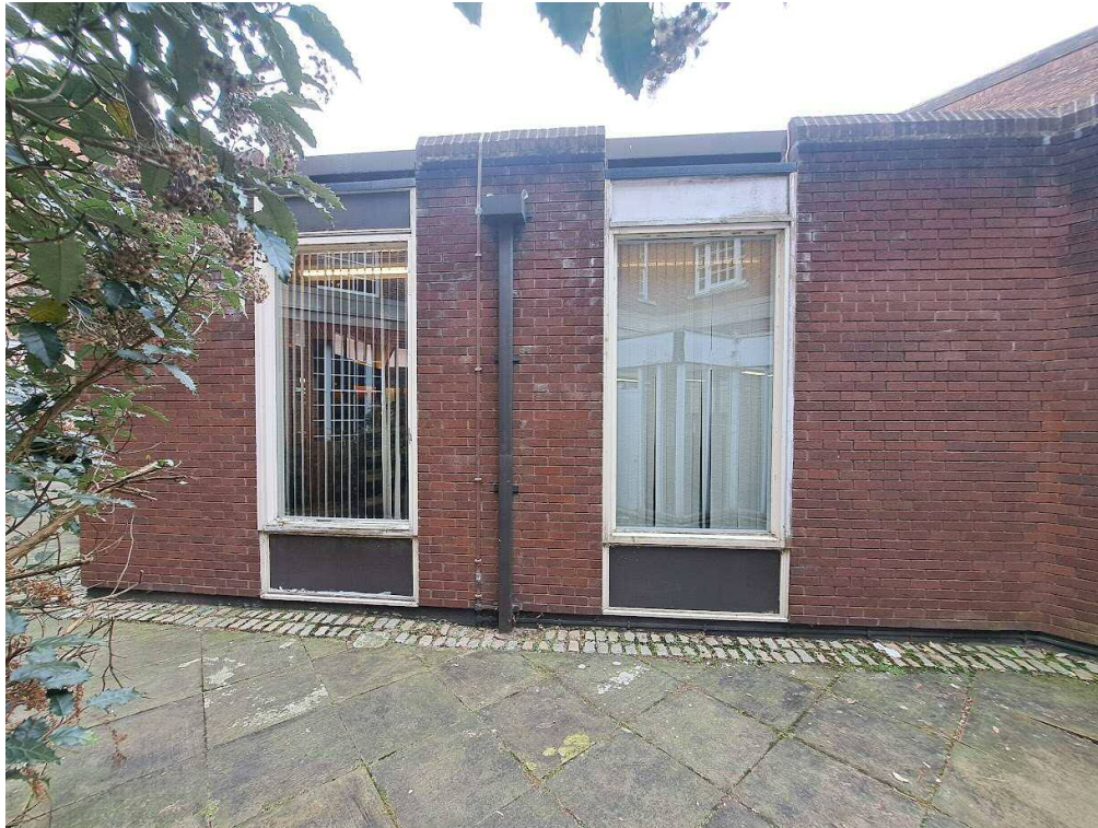
Photo 1. Windows W1 and W2.
