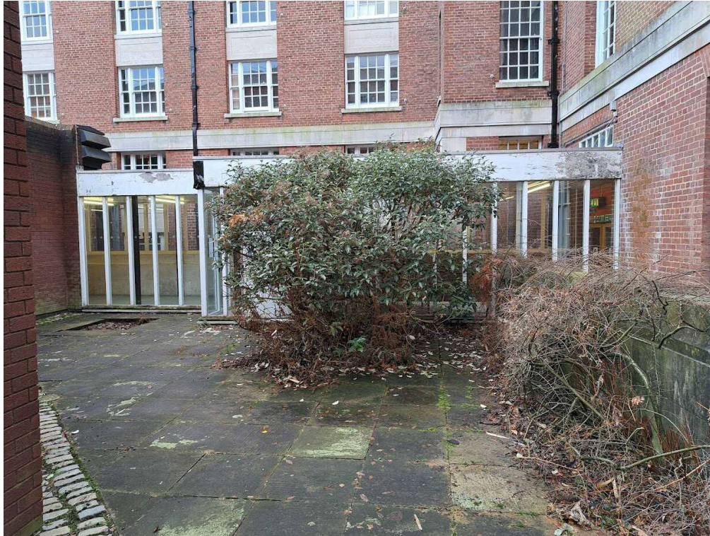
Photo 12. Fire door D4 in Elevation 5.
