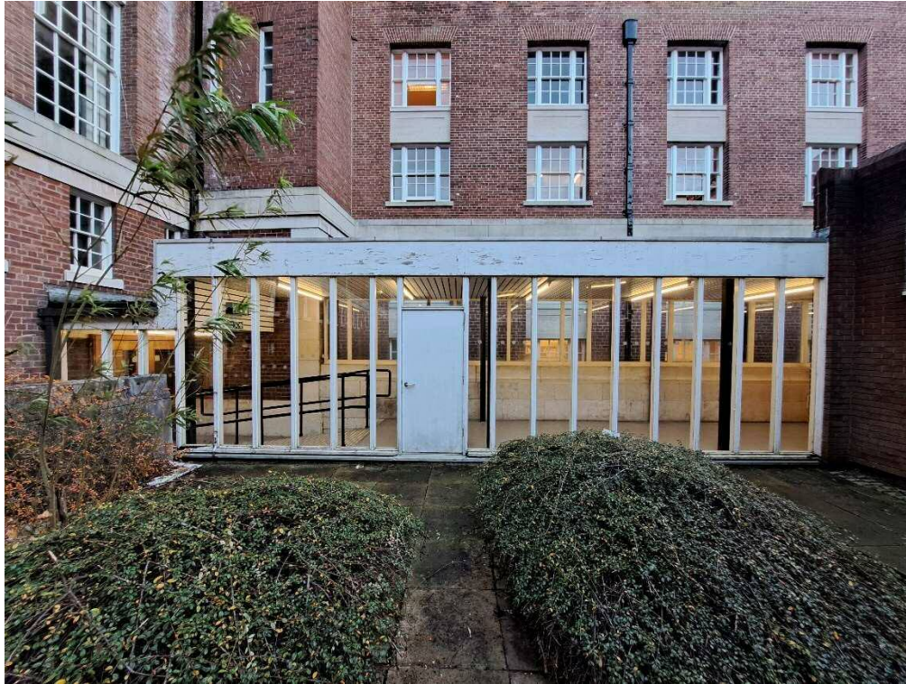
Photo 10. Fire door D3 in Elevation 5.
