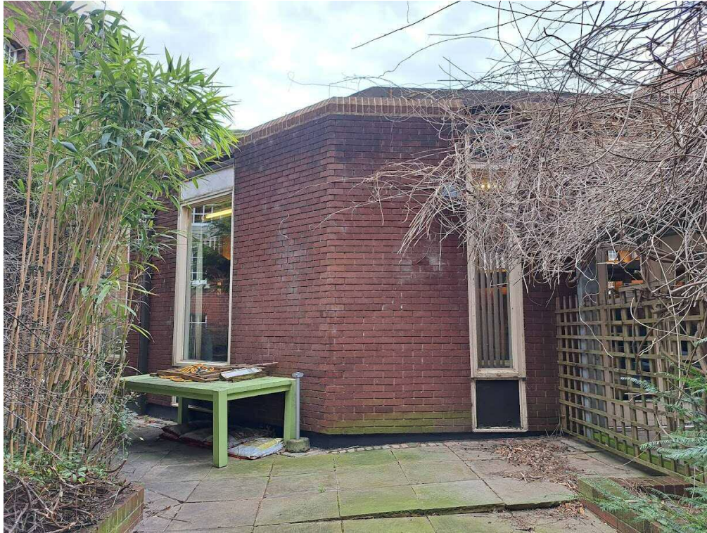
Photo 6. Windows W8 and W9.
