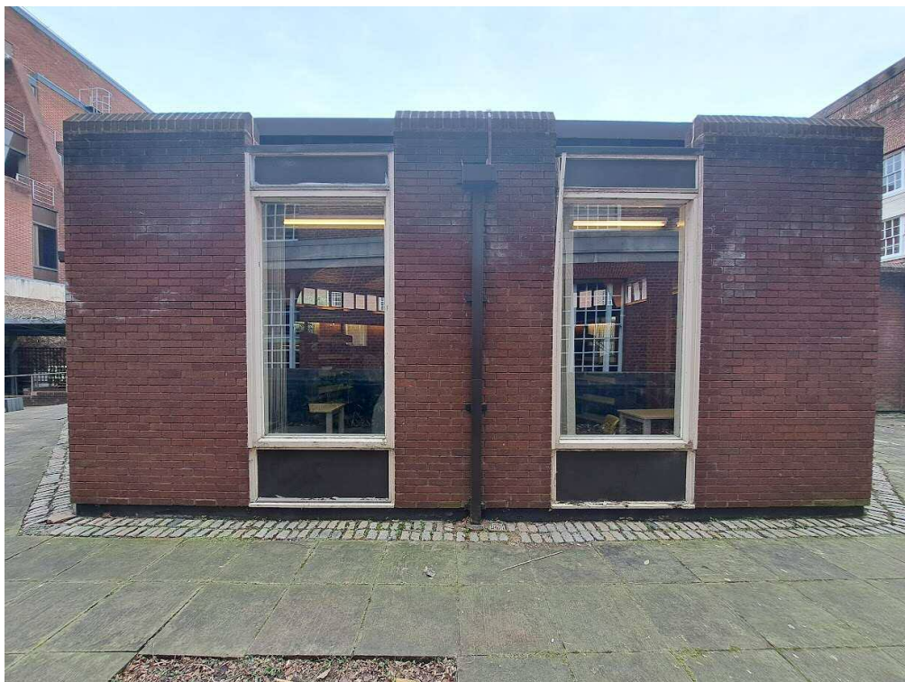
Photo 2. Windows W3 and W4.
