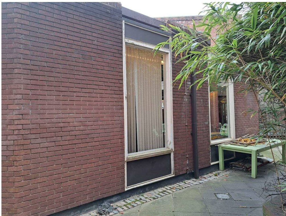
Photo 7. Windows W9 and W10.
