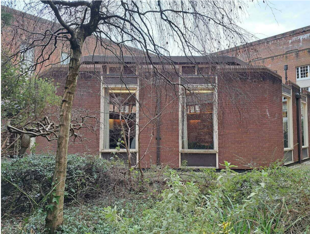
Photo 3. Windows W5 and W6.
