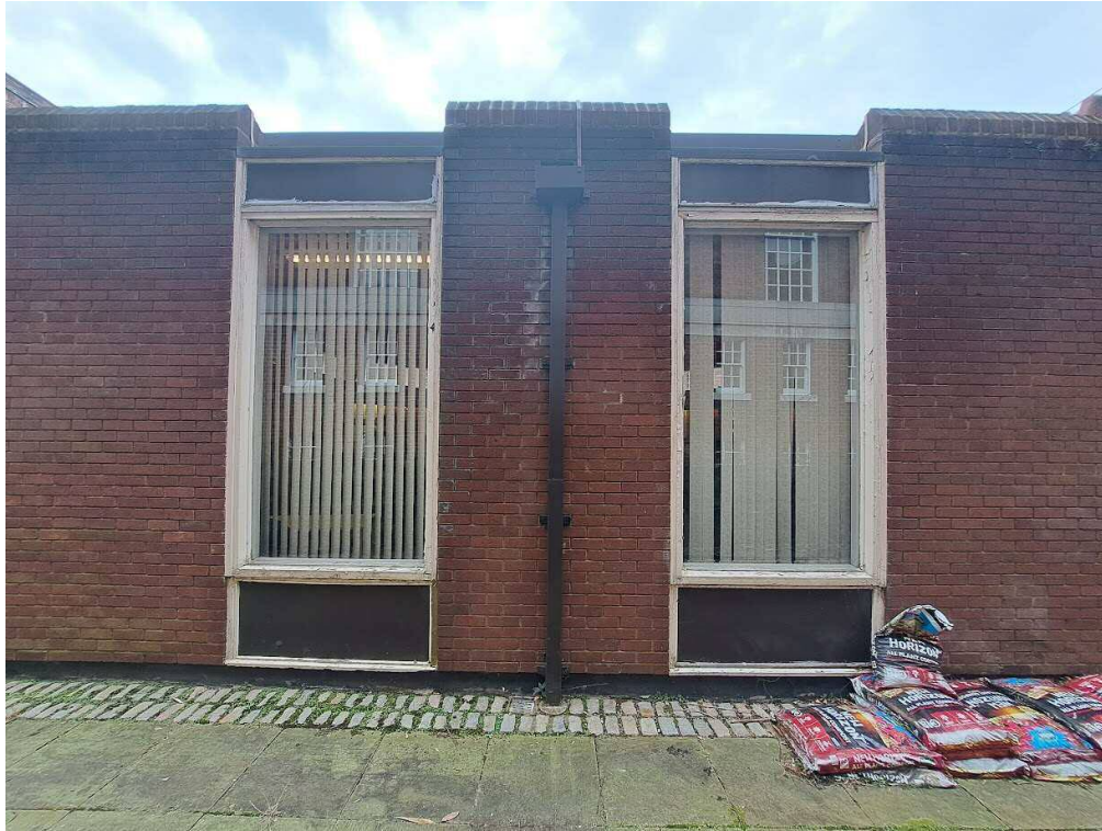
Photo 8. Windows W11 and W12.
