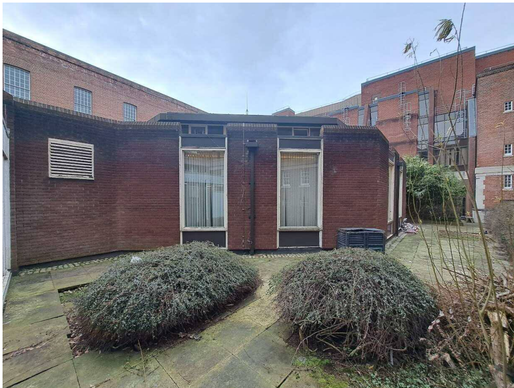
Photo 9. Windows W13 and W14.
