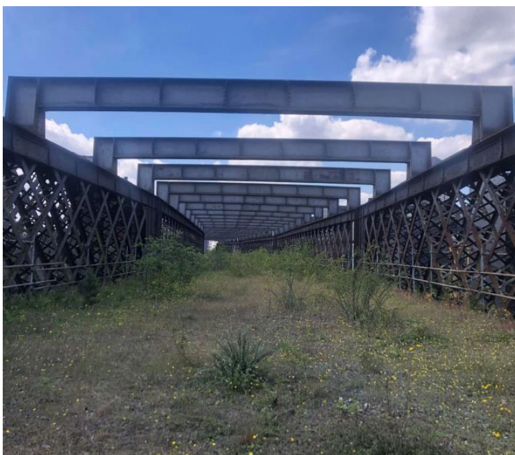
Figure 2 – Existing vacant viaduct (Phase 2)
