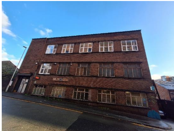
PLATE 1 SHOWING SOUTH-WEST ASPECT OF BUILDING
