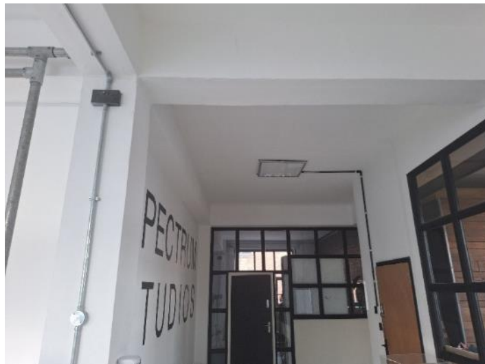
PLATE 7 SHOWING INTERNAL 2ND FLOOR
