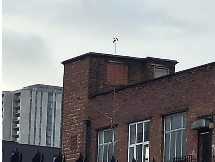
PLATE 6 SHOWING ROOF FROM GROUND LEVEL
