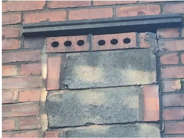
PLATE 4 SHOWING FILLED IN WINDOW
