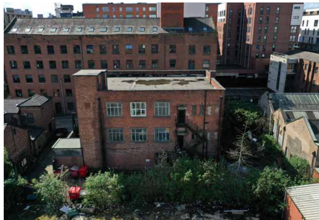
Figure 4.2 The rear, east elevation of the Site. Beehive Mill is visible behind the Site and large-scale modern developments are located in the background.
