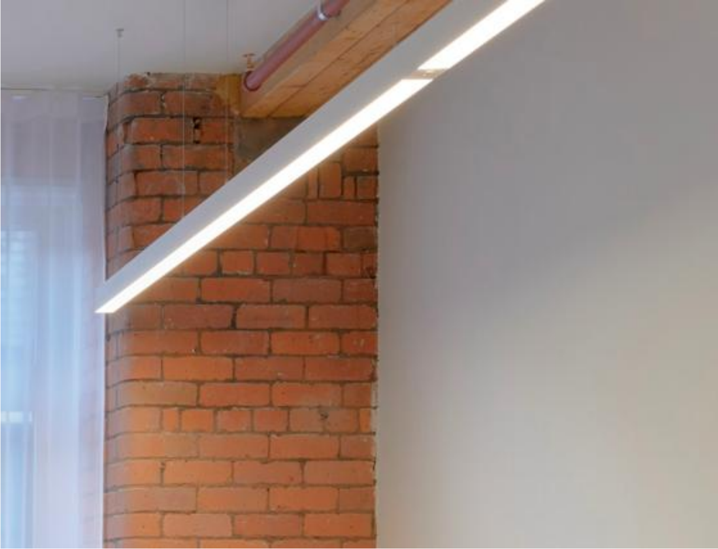
Photograph of an existing contemporary plasterboard stud partition abutting an exposed masonry wall pier as part of the consented works under LBC application (130043/LO/2021). The partition is neatly scribed to the inconsistent brick faces.
