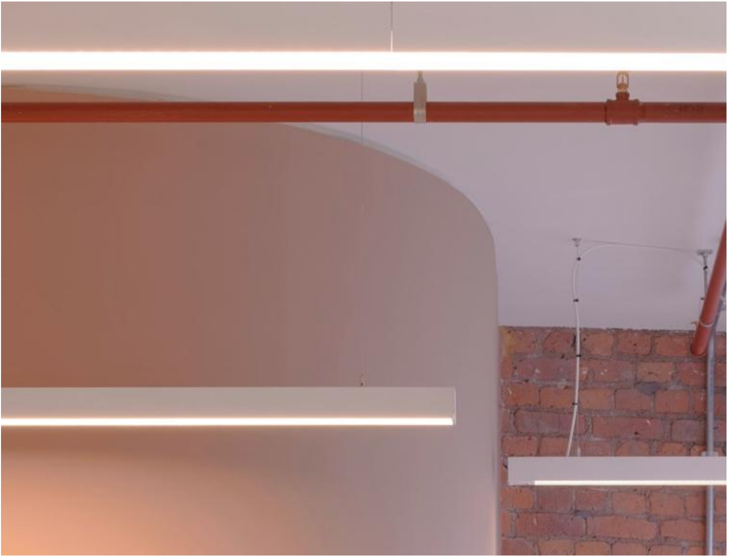
Photograph of an existing contemporary plasterboard stud partition abutting an underdrawn lath & plaster ceiling as part of the consented works under LBC application (130043/LO/2021). The deflection head detail is visible.
