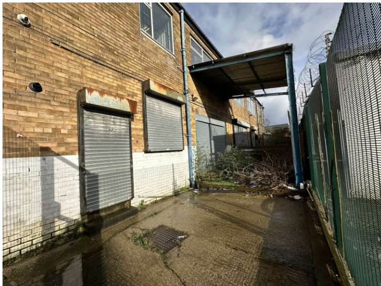
Figure 3. Existing Curtilage at the Rear 2025
