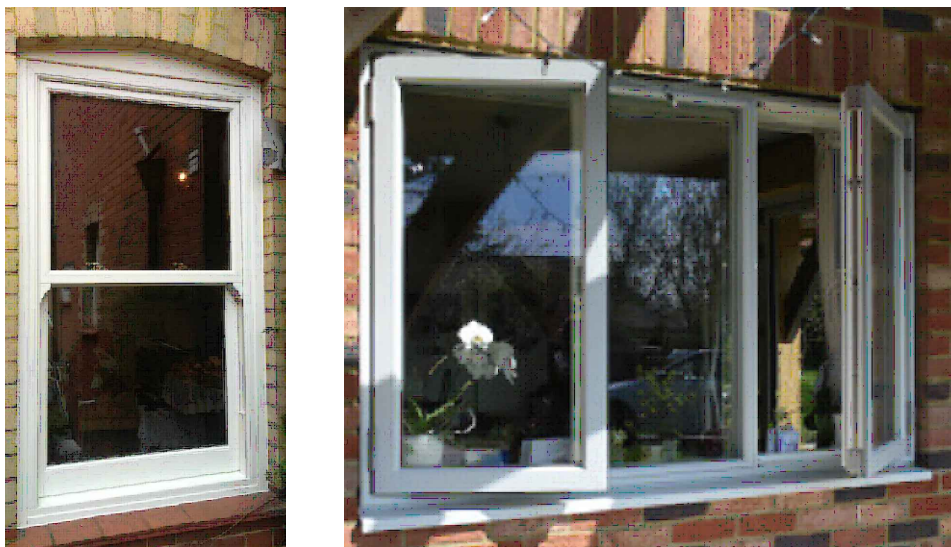
UPVC Double Glazed Window UPVC Sliding Sash Replacement For Existing UPVC Side Hung At Roof Level Colour White
