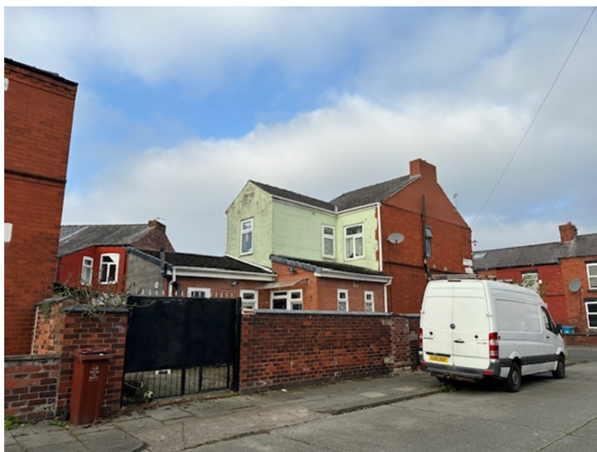
Side and rear elevations of 4 Highfield Road
