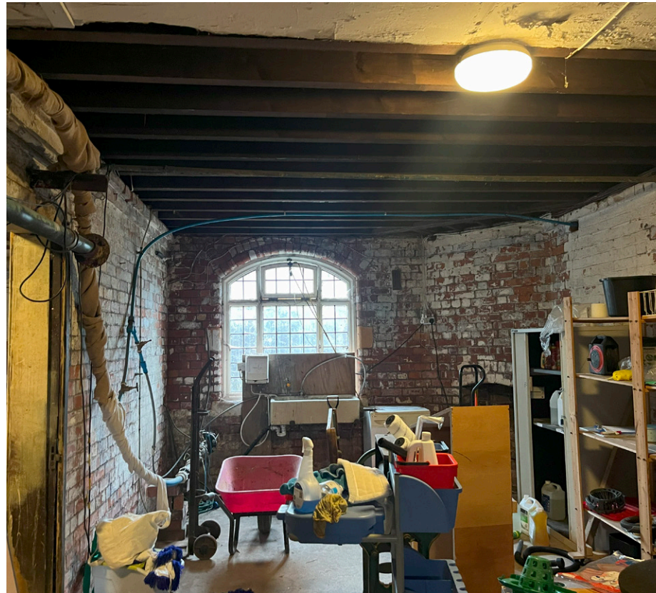
Figure 3 Below: Basement Spaces to be Subject to Asbestos Removal
