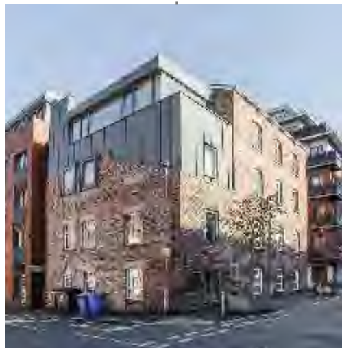
Former warehouse on Simpson St / Sharp St junction
