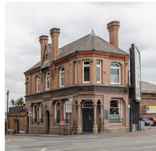
Marble Arch Inn public house on Rochdale Road
