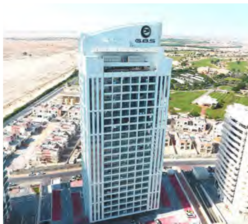
245 Apartments - GBS Residences - UAE - Dubai
